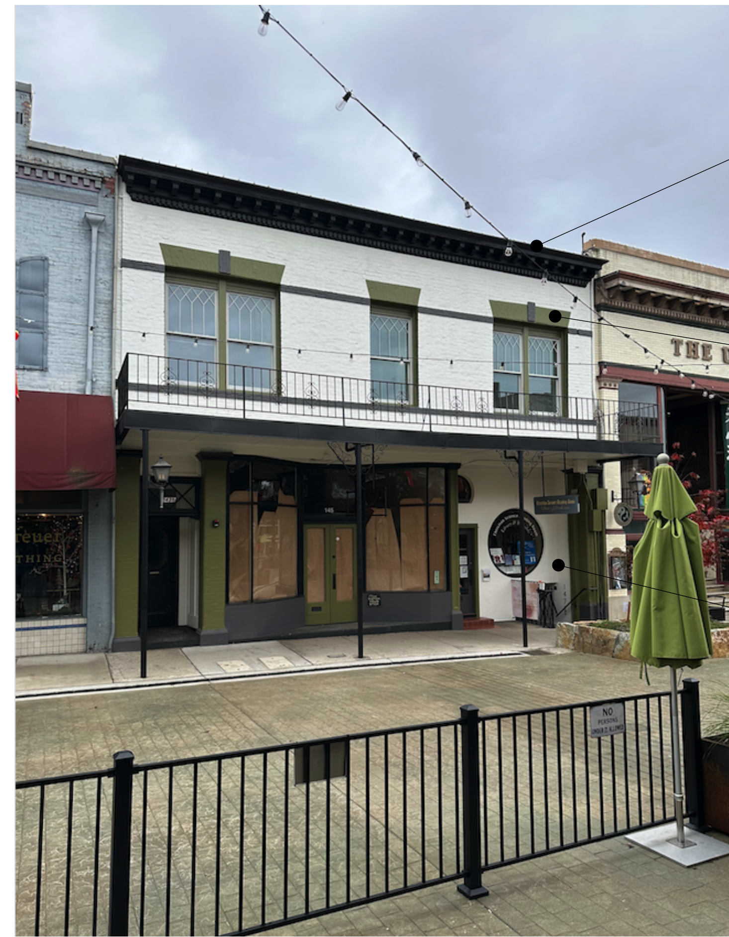
145 MILL STREET VIEW
