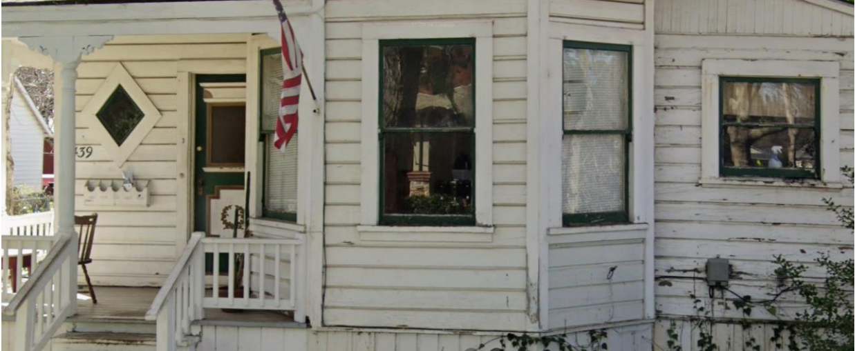
2024 Google Maps image capture (lower level windows)
