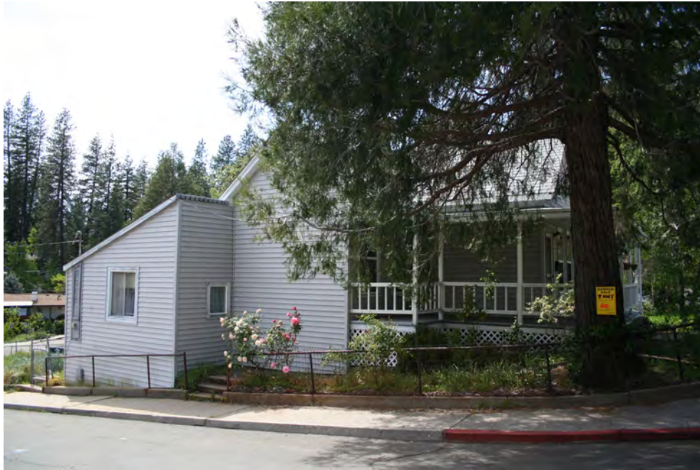
View looking southwest at the residence. Note the shed roof addition in the rear.
