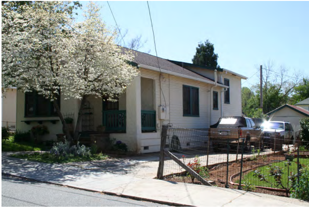
View looking southwest at the north elevation of the house. Note the rear shed roof addition.
