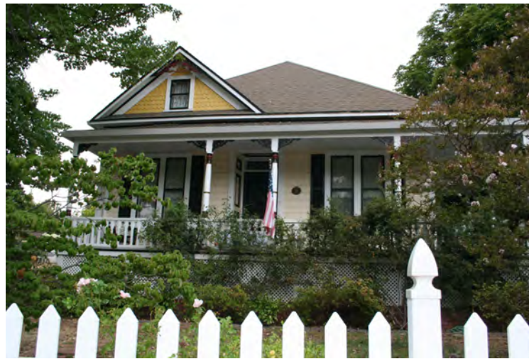
View of the front facade looking west.
