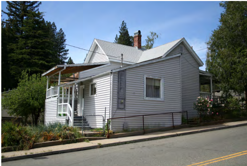
View looking northwest at the residence. Note the addition of decks in the rear of the house.
