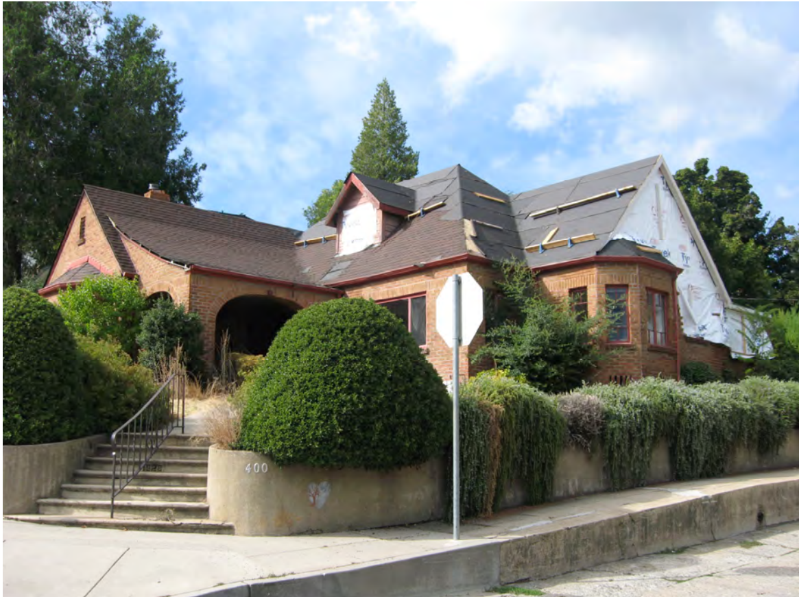
View looking northwest at the residence under rehabilitation following the fire.
