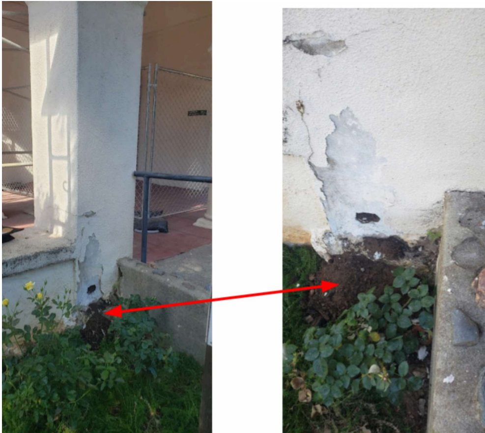
Figure 3- Wood debris from inside the easternmost column
