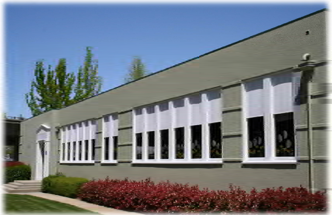
Use of a repeating ribbon type window in a Grass Valley school building.
