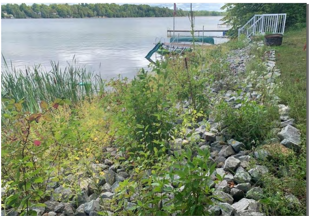
VEGETATED ROCK SLOPE PROTECTION https://watersheds.ca/wp-content/uploads/2022/06/RVCAs-Vegetated-Rip-Rap-handout.pdf
