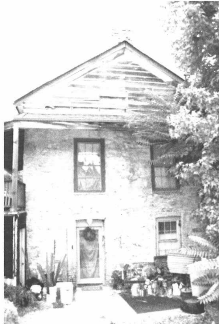
Photograph looking north at the lower story (south elevation).
