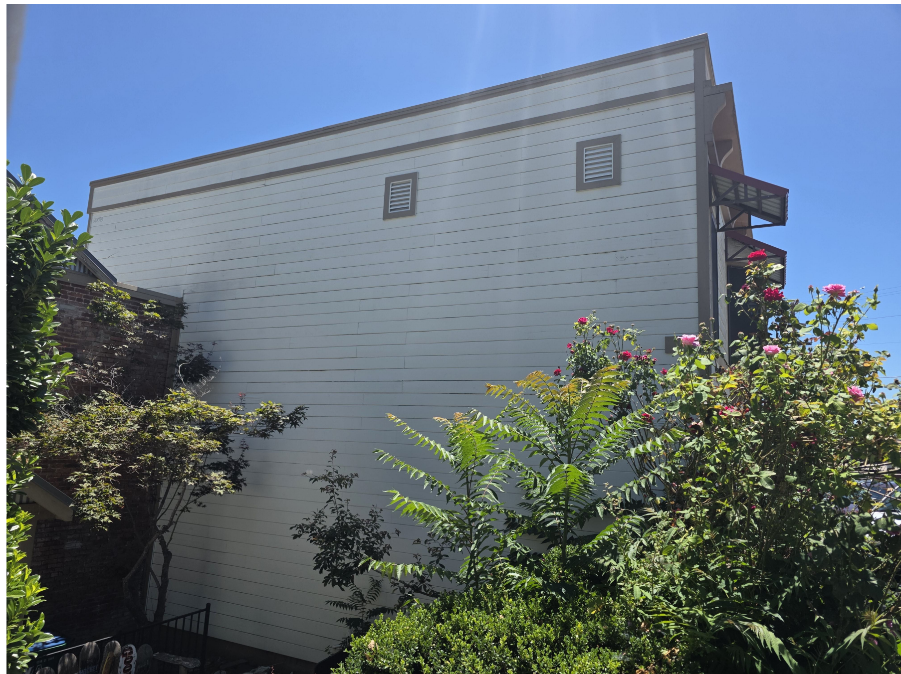
NOTE: PICTURE OF EXISTING NORTH FACADE
