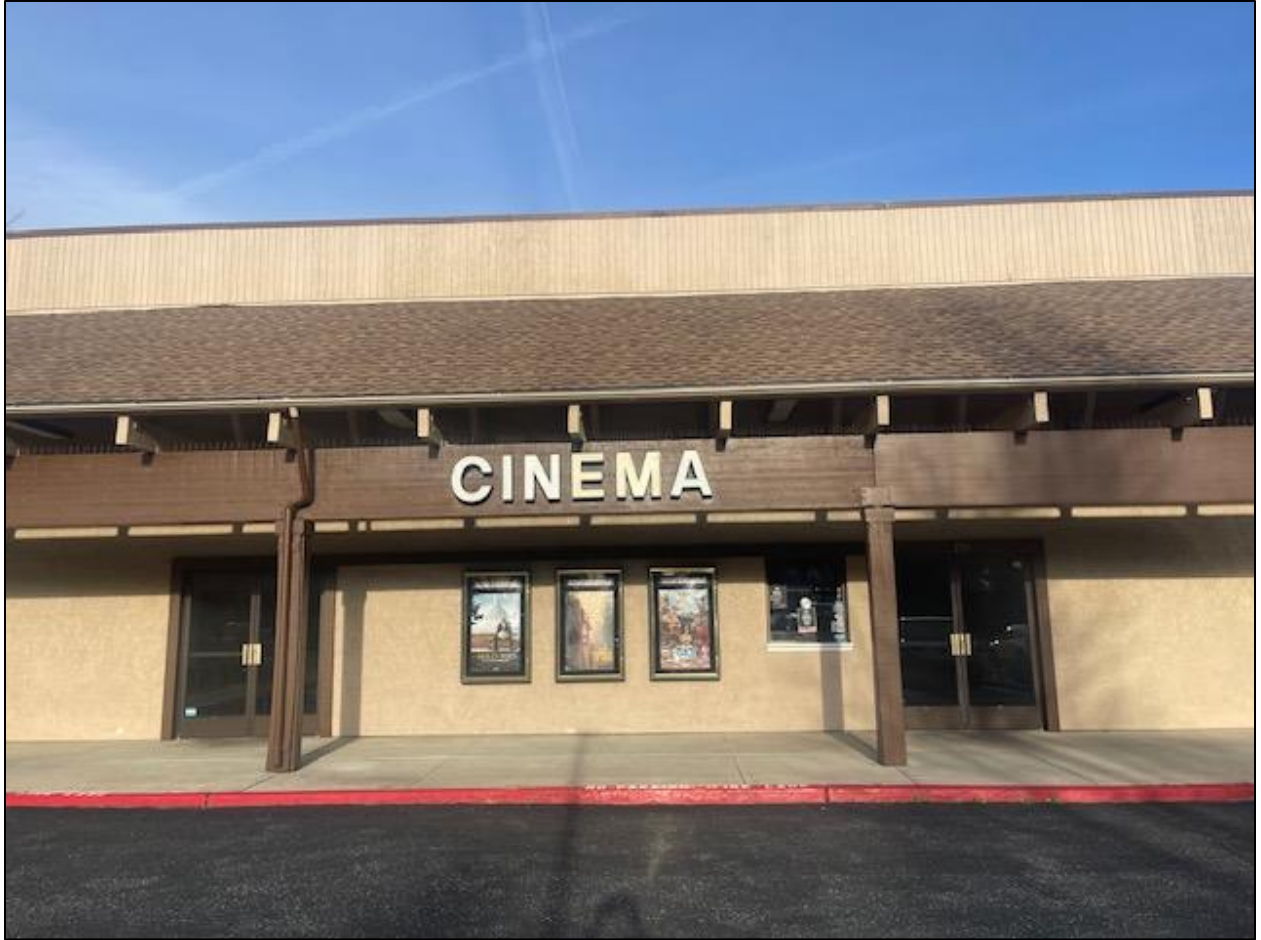
Existing Building Face
