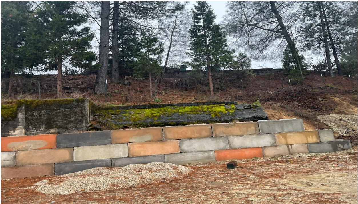
Photo 4: Photo looking south from the Project area with an existing retaining wall and some pine trees upslope outside of the Project area. Trees are outside Project fenceline.
