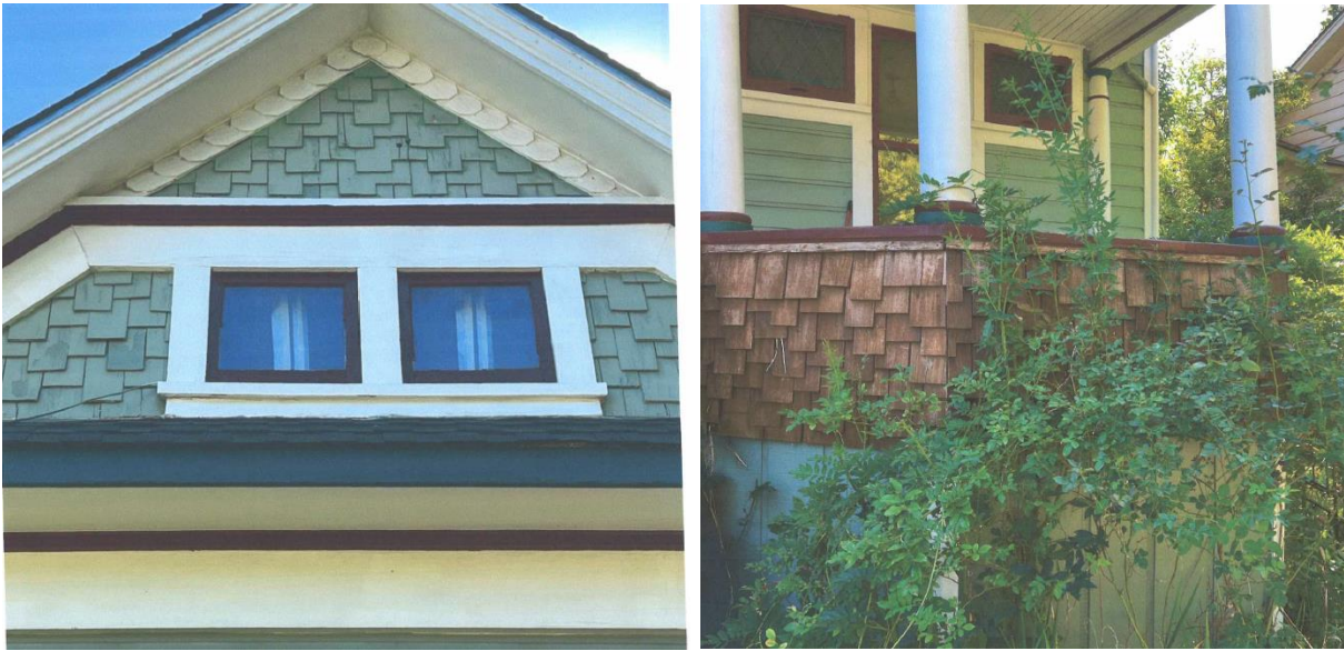
Existing Shingled Siding at 257 South Auburn Street
