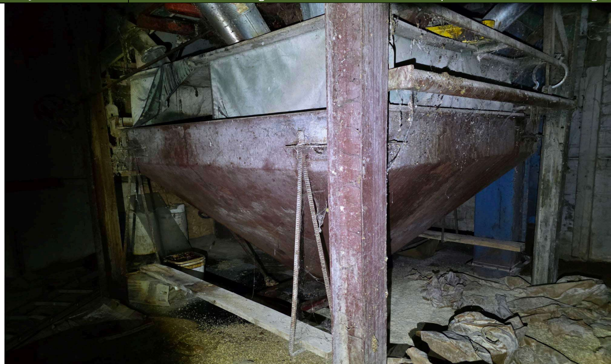
Photograph 30 Date: April 14 th , 2026 Direction: Southwest Subject: Seed bag filling area in the eastern portion of the Site building, fed from the grain silos east of the Site building. Staining and various empty bags present.
