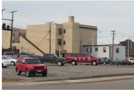
The view shows Block 19 from 1st Avenue East. The east half of Block 19 is a parking lot. The “backs” of these buildings do not cover an attractive face or clear points of access. Power lines should be buried as part of redevelopment.
