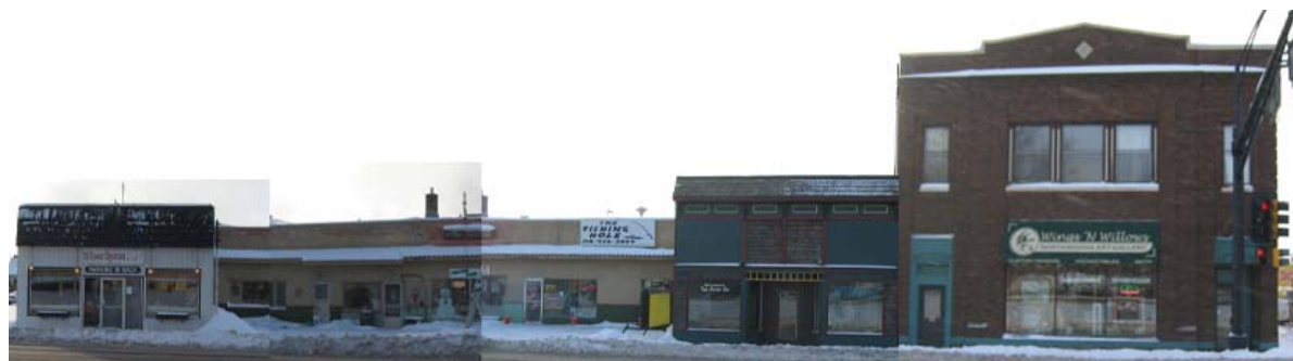
Existing building on Block 37 viewed from Highway 2.
