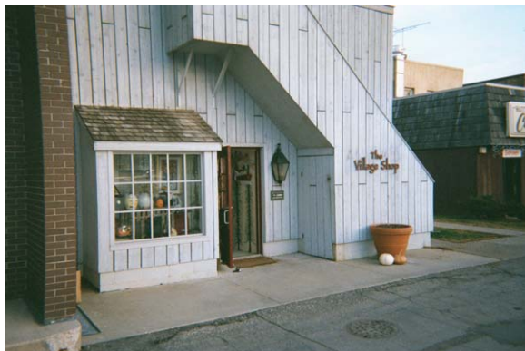
Rear building entrance in Hutchinson
