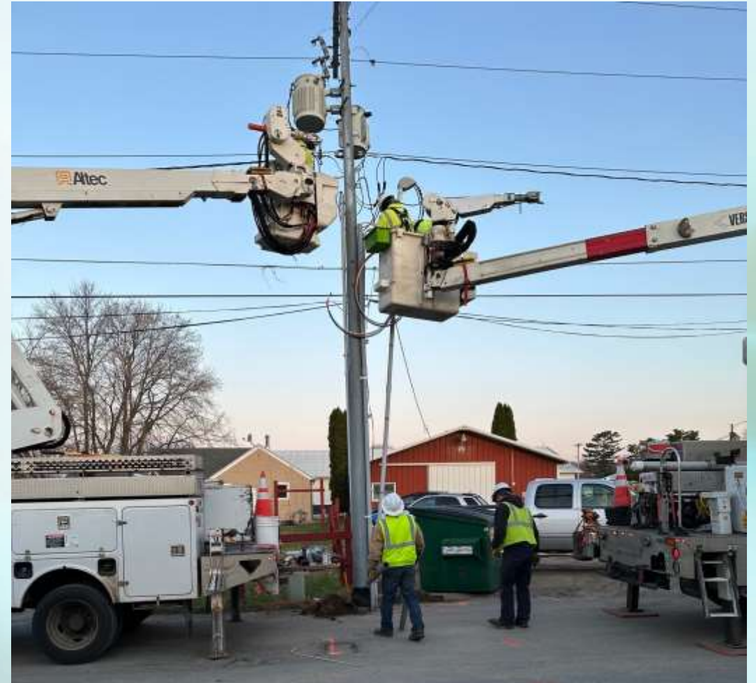
Early Morning Outage for Service Upgrade.
