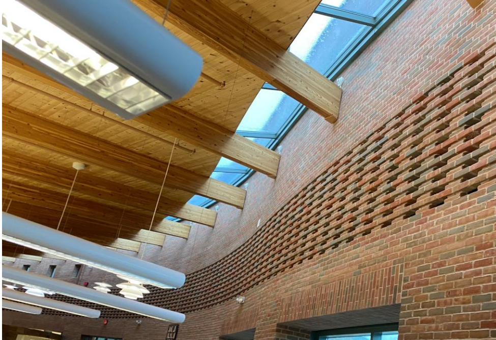
Photograph 20 – Interior view of skylight assemblies.
