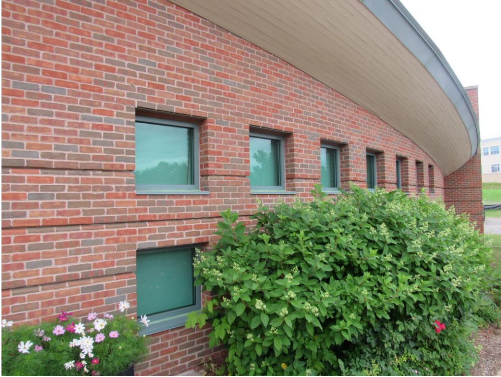
Photograph 12 – Typical lintel details at masonry window fenestrations.
