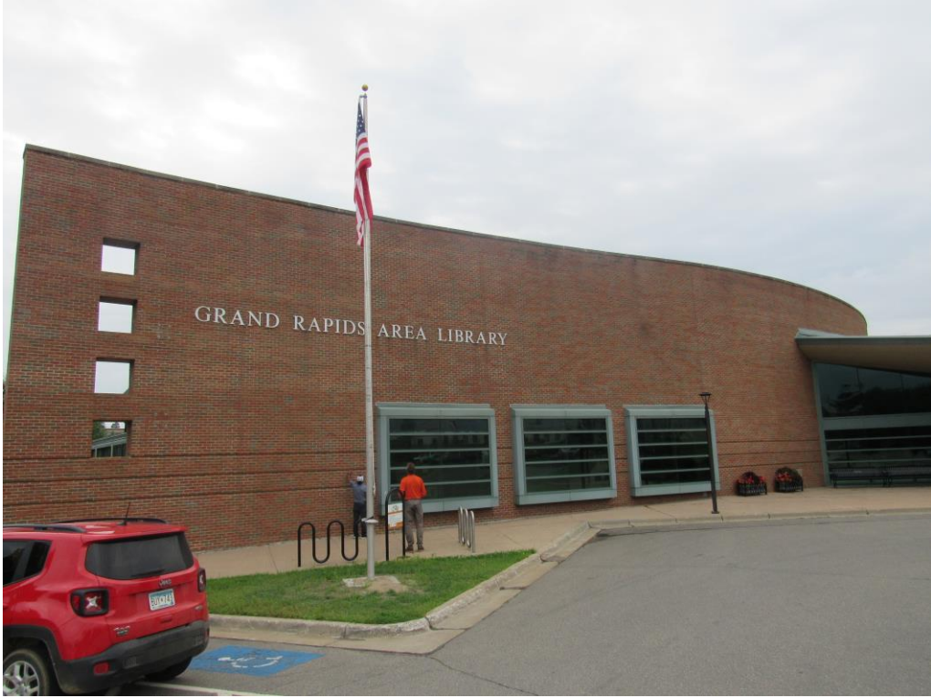
Photograph 1 – The east (front) elevation of the library building.
