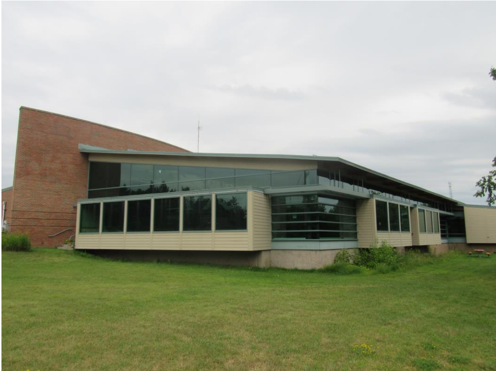
Photograph 2 – The west elevation of the library building.
