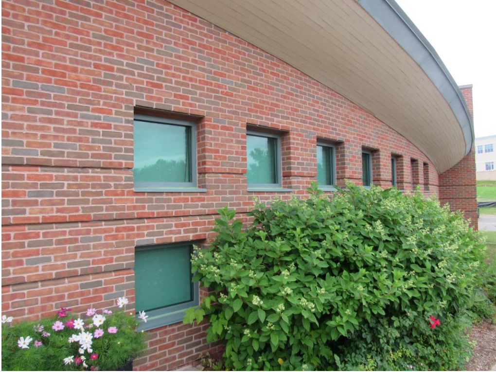
Photograph 12 – Typical lintel details at masonry window fenestrations.
