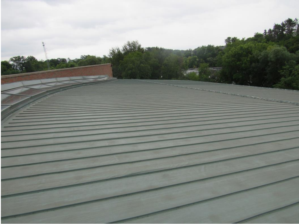
Photograph 28 – Roofing at the south roof elevation.
