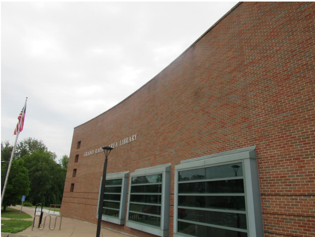
Photograph 11 – Typical masonry conditions at the north elevation.
