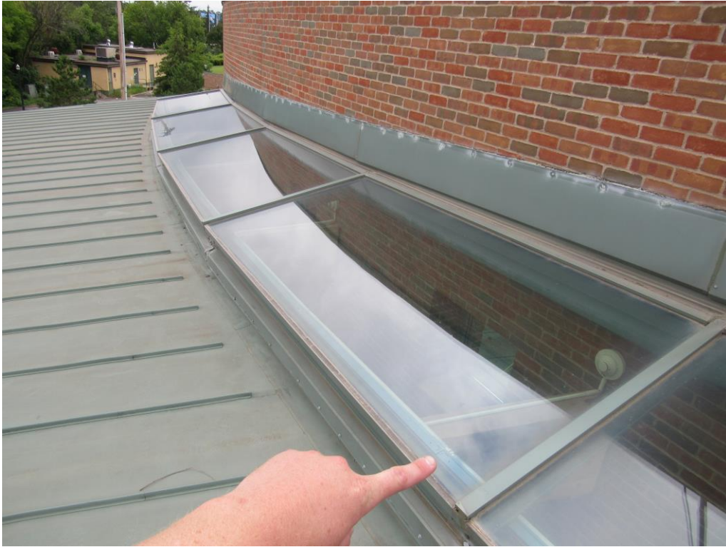
Photograph 10 – Water testing location at the skylights.
