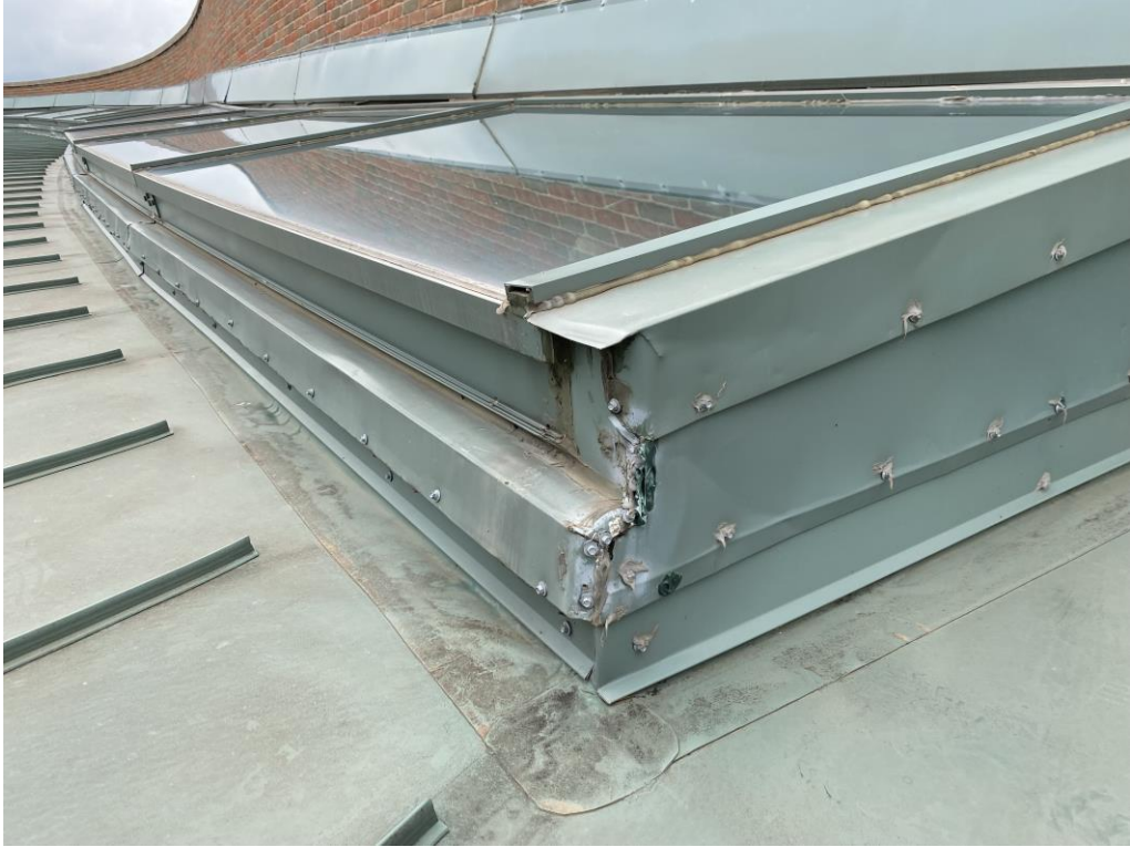
Photograph 22 – Repairs at the skylight joints.
