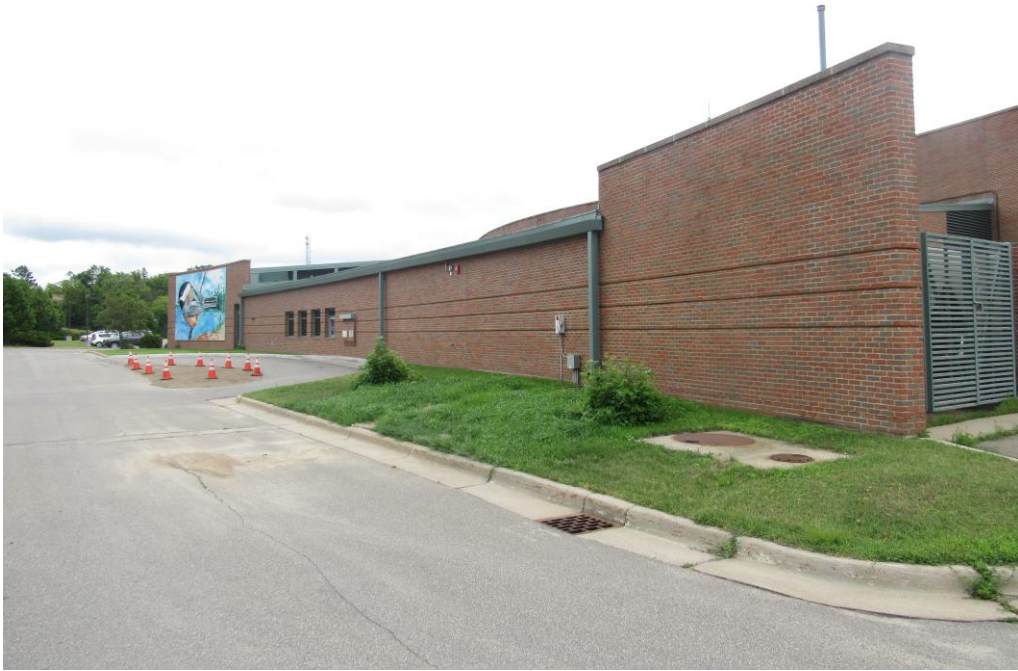
Photograph 3 – The north elevation of the library building.
