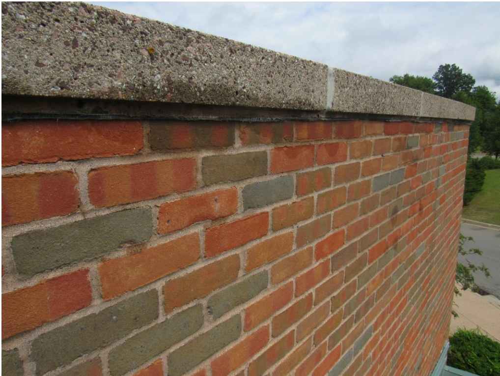
Photograph 15 – Wall cap details showing flashing conditions.
