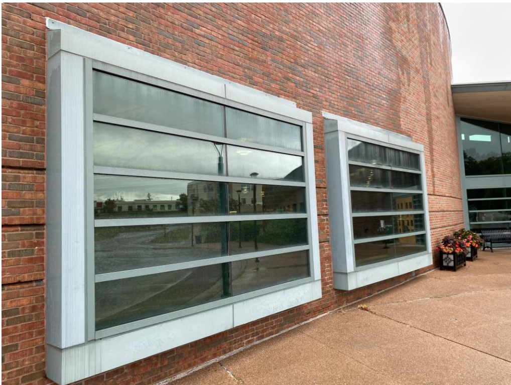
Photograph 4 – Bumpout window assembly near the main entrance.
