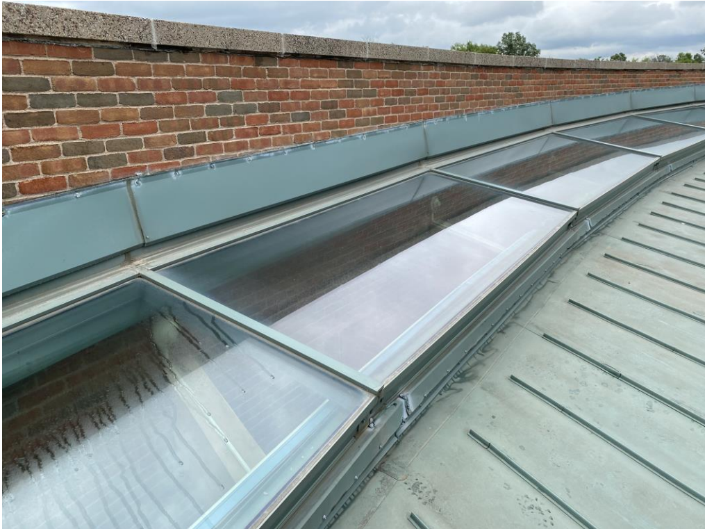
Photograph 19 – Skylight assembly at the roof.
