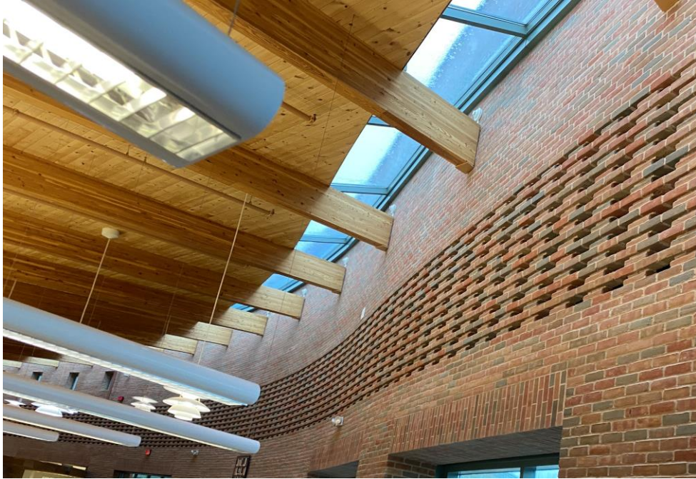
Photograph 20 – Interior view of skylight assemblies.
