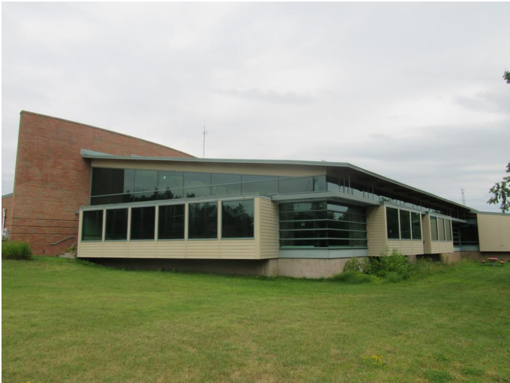
Photograph 2 – The west elevation of the library building.
