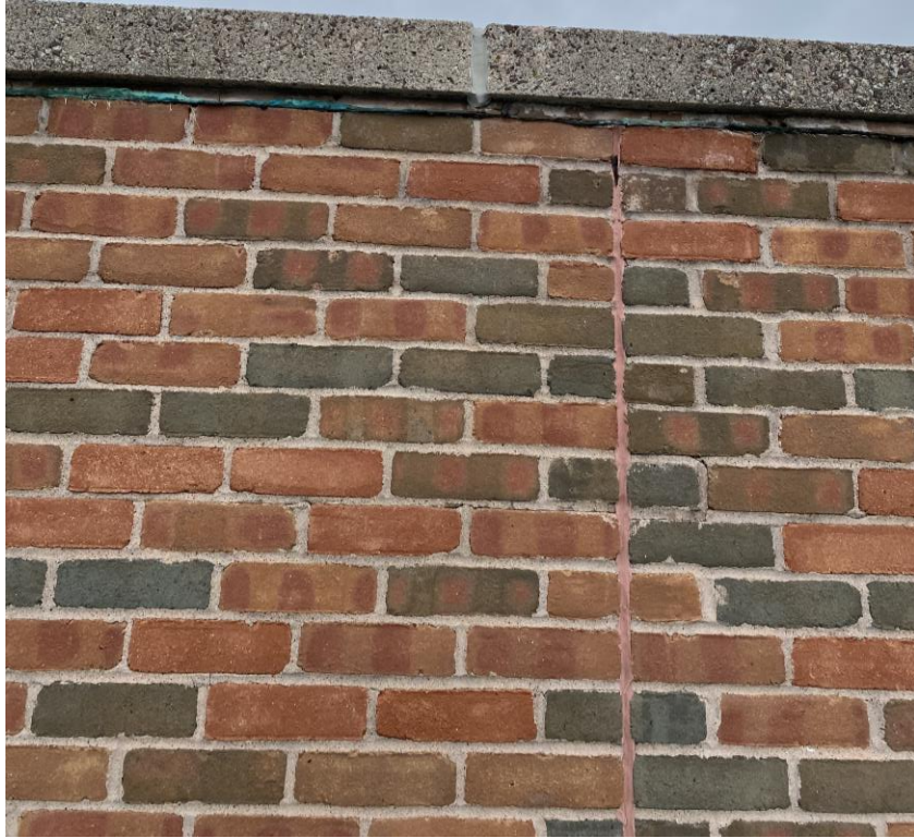
Photograph 26 – Sealant at masonry joints.
