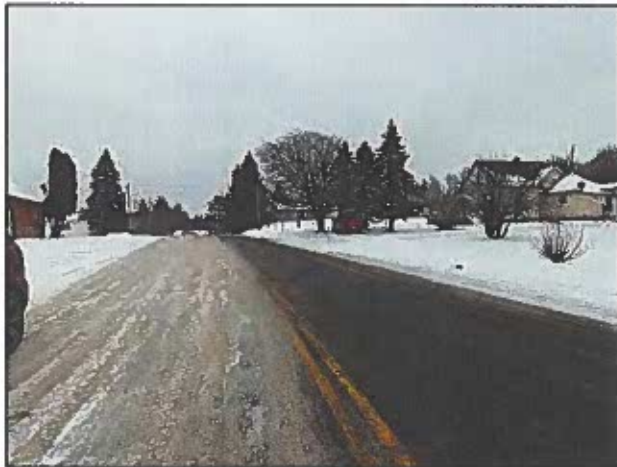
Looking northerly along NE 10 th Avenue from U.S. Highway 2 E (TH 2)
