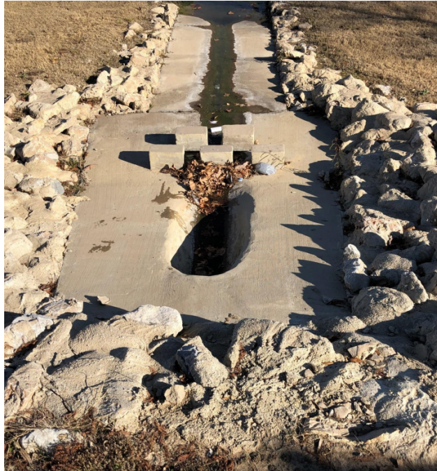
Photo 3: Downstream view of the structure and apron
