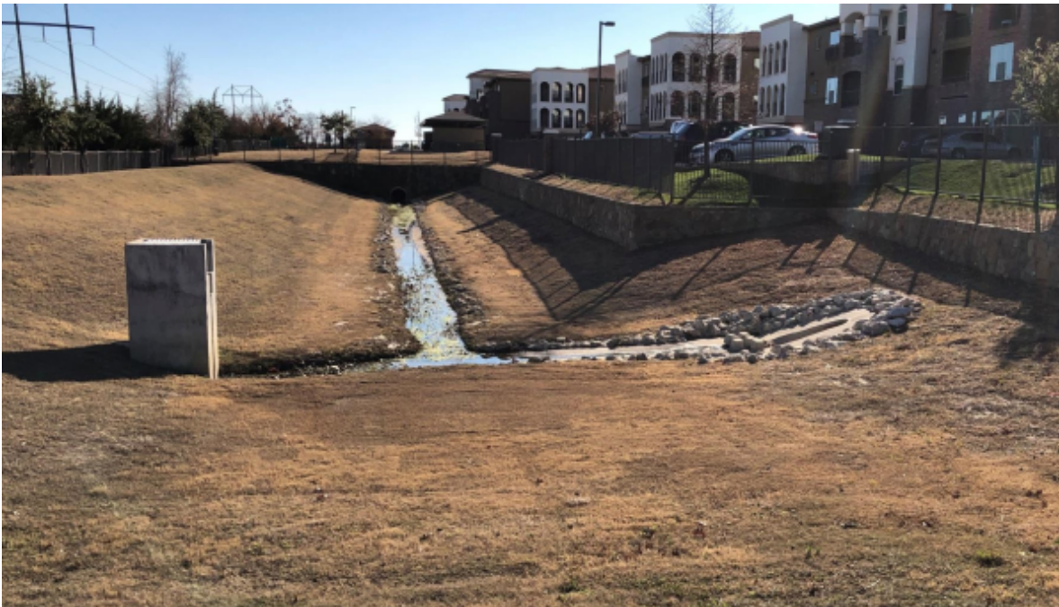
Photo 4: Downstream view of the channel that receives flow from structure
