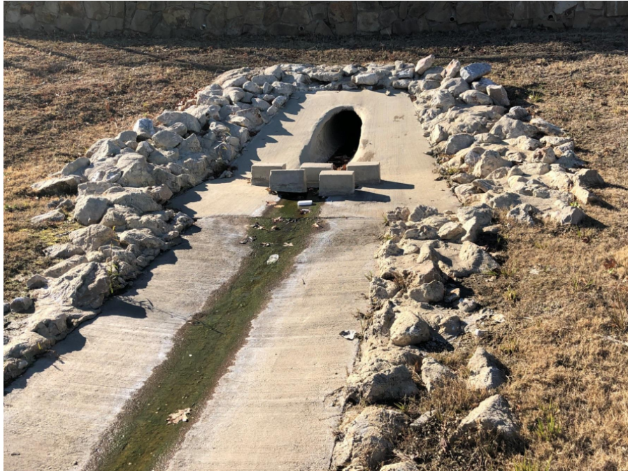
Photo 5: Upstream view of structure (include headwall, side slopes and apron)
