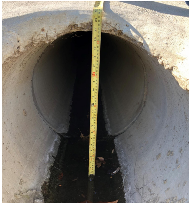
Photo 6: Focused upstream view of structure
