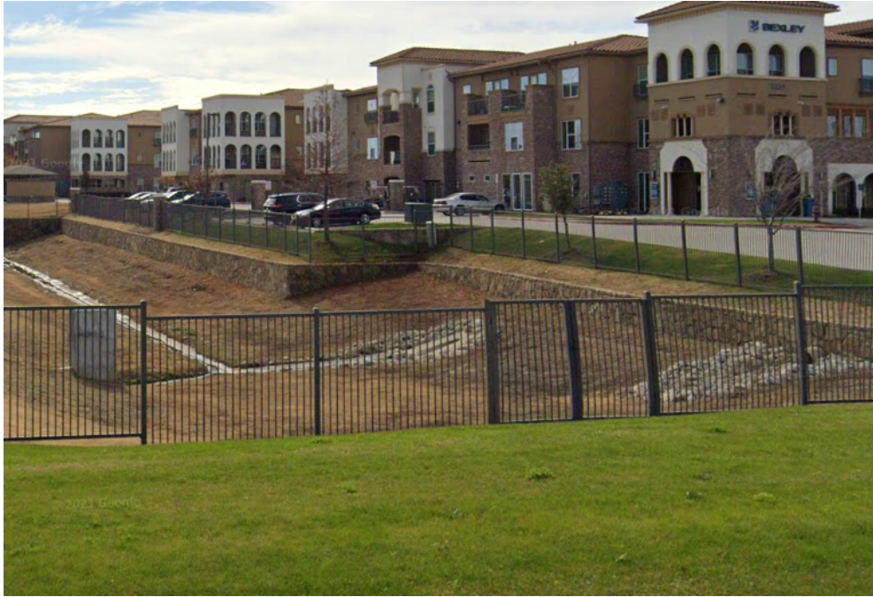
Photo 1: Area view of the structure
