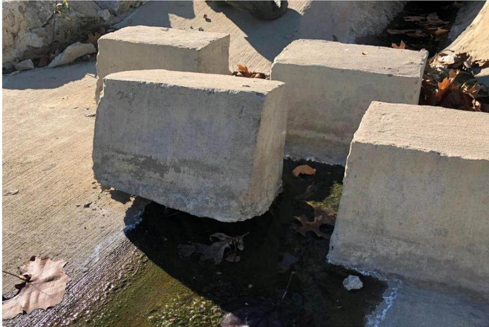
*Photo 7: Any additional photos to support inspection (example, loose baffle block)*
