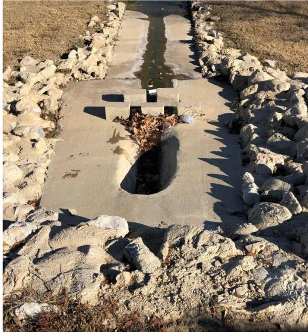
*Photo 3: Downstream view of the structure and apron*
