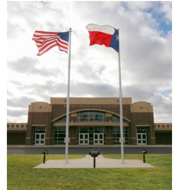
Brownwood High School Renovations
