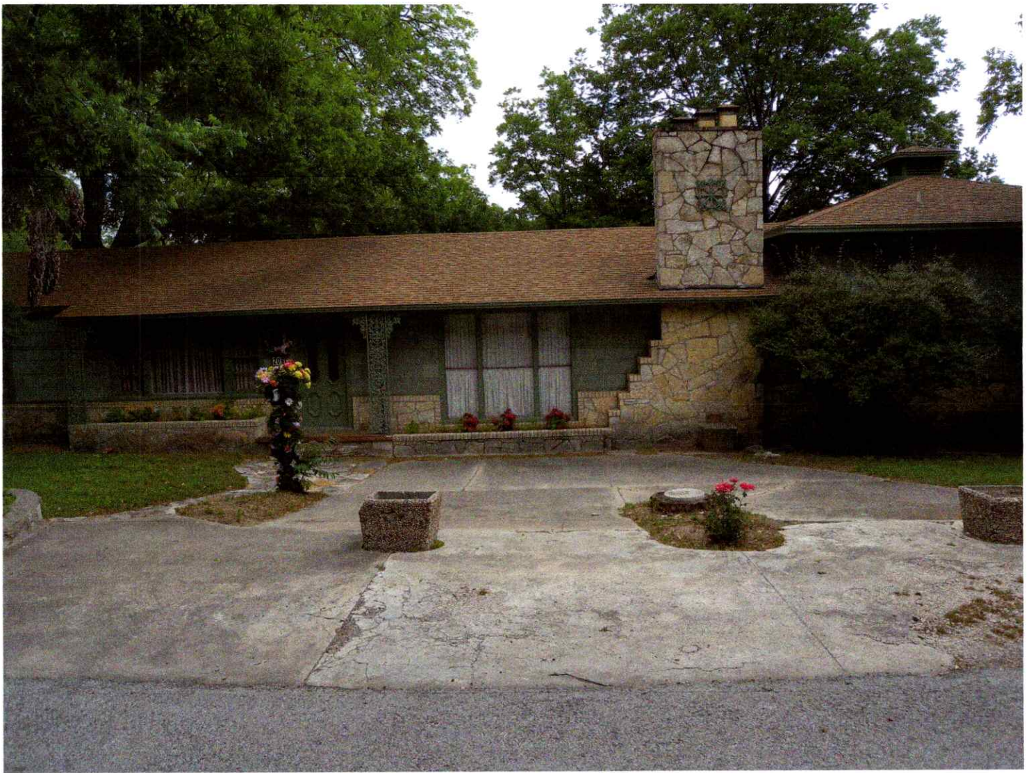
Glen Rose Historic Resources Survey, Site 39 (roll 4, exp. 28), residence, 206 Northeast Vine Street, southeast to front of house showing what appears to be the concrete drive that served an earlier garage before the structure was expanded with a combined split-level garage/living area at the southwest end.
