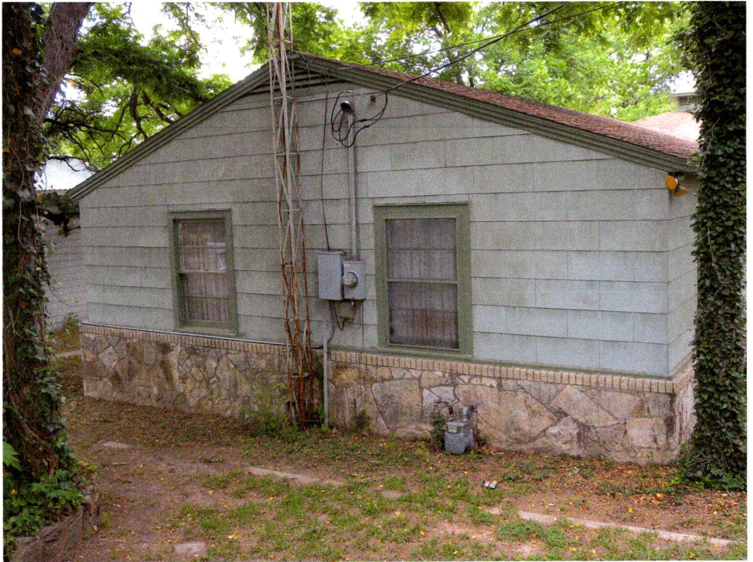
Glen Rose Historic Resources Survey, Site 39 (roll 4, exp. 30), residence, 206 Northeast Vine Street, south to northeast side showing stone veneer at base of wall, asbestos siding on upper portion of wall, and the lower portion of the historic television antenna.
