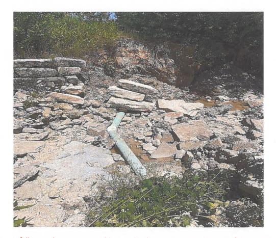
The recent rainfall caused an erosion problem in the drainage area to the east of the waste water treatment facility. About 20 linear feet of 8" plastic sewer main was exposed by the white-water rapids. We were able to remove the boulders from the top of the pipe, and then excavate around the pipe, without damaging anything. The pipe was then completely encased in 10 yards of concrete.
