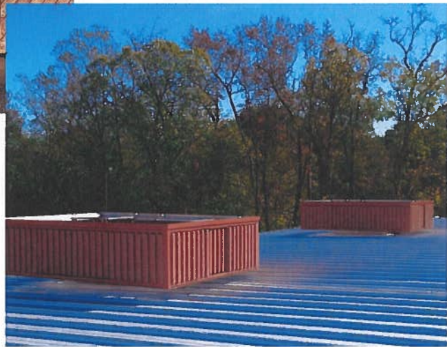
Rooftop Equipment Screening Sample
