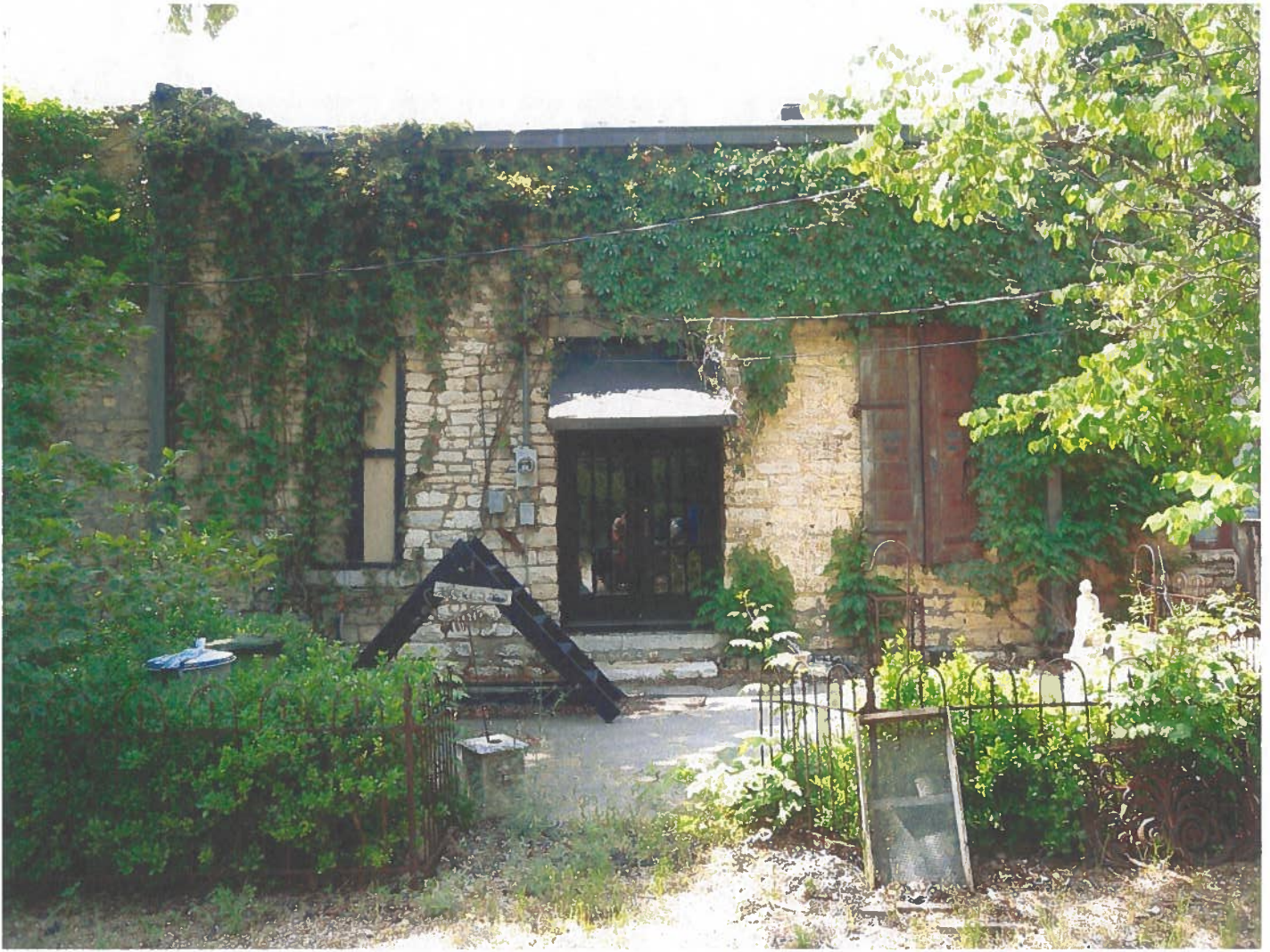
Glen Rose Historic Resources Survey, Site 58 (roll 6, exp. 28), J.R. Milam Company, 103 Southwest Barnard Street, northwest to rear.
