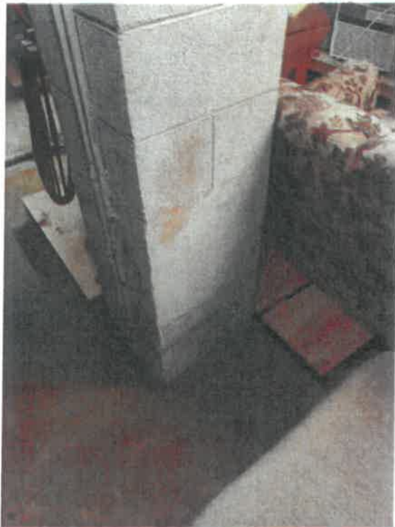
Photo 4: Patched masonry column (typ)
