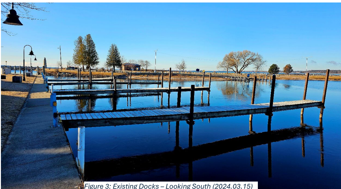
Figure 3: Existing Docks – Looking South (2024.03.15)
