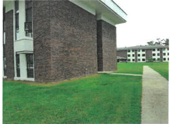
SOUTH ELEVATION OF SUBJECT BUILDING
