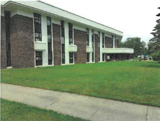
SOUTHEAST ELEVATION OF SUBJECT BUILDING
