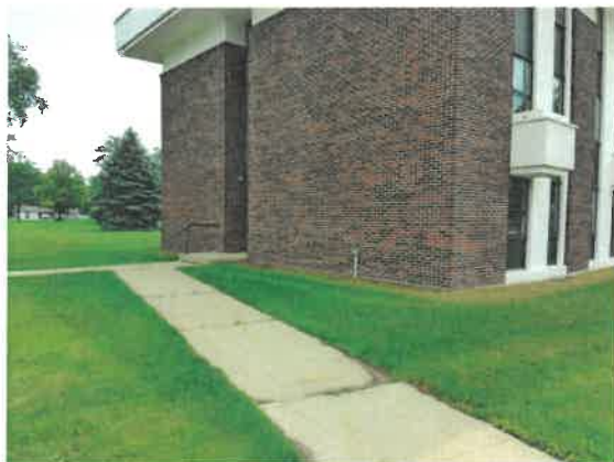
NORTH ELEVATION OF SUBJECT BUILDING
