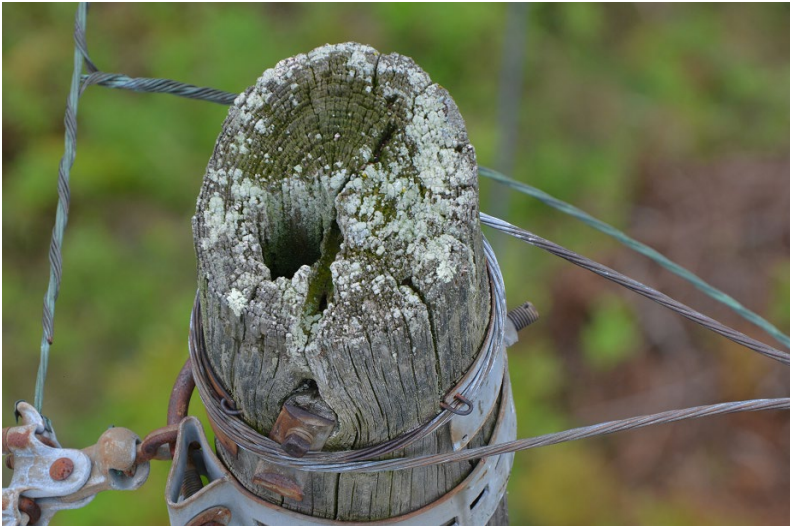
Examples of rotted pole tops
