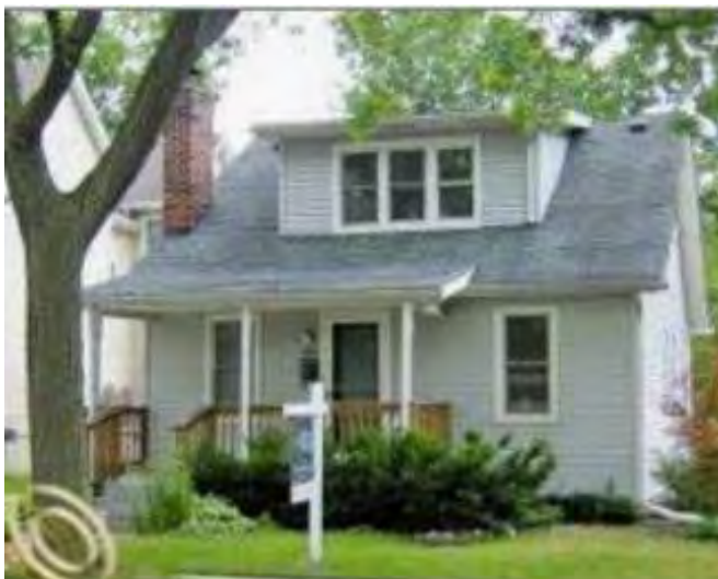
Figure 10.2 - Shed dormer, with a single, inclined roof.
