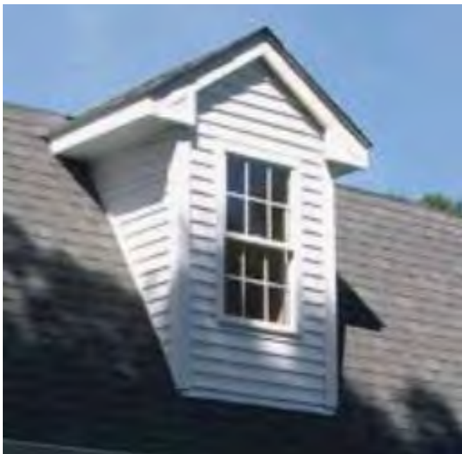
Figure 10.1 - Dog house dormer, with gable roof
