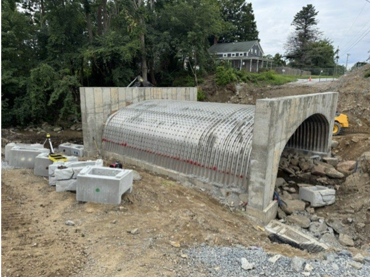
Bridge construction: arch installation and site preparation
