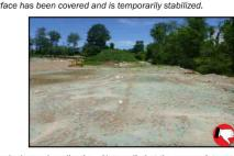
Poor hydroseed application. Not applied at the appropriate rate, soil not prepared, and very little mulch component in mix.
