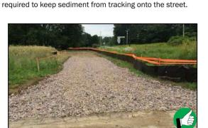
Good stabilized construction access. Adequate width to accommodate construction traffic and prevent mud tracking offsite. Ensure that the pad is 8 inches deep and 40 feet long.
