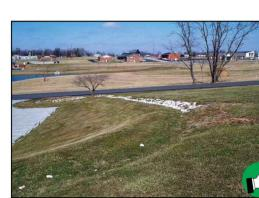
Good construction, seeding, and stabilization of diversion berm. Note that liversion ditch is lined with grass on flatter part of slope, and with rock on
