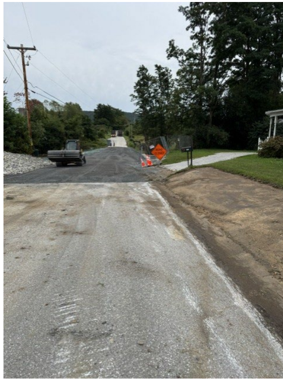
Bridge finished waiting on paving
