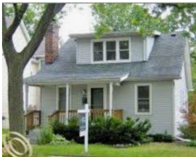
Figure 10.2 - Shed dormer, with a single, inclined roof.
