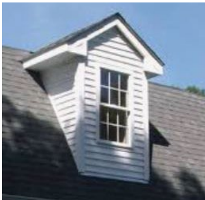
Figure 10.1 - Dog house dormer, with gable roof
