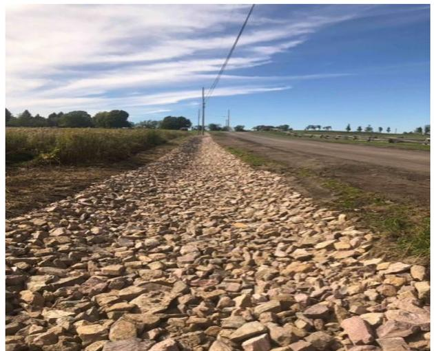
*Figure 2.3: This new stone lined ditch on Kibbe Point Road was funded by Grants In Aid in 2022 and will reduce erosion and improve stormwater infiltration.*
