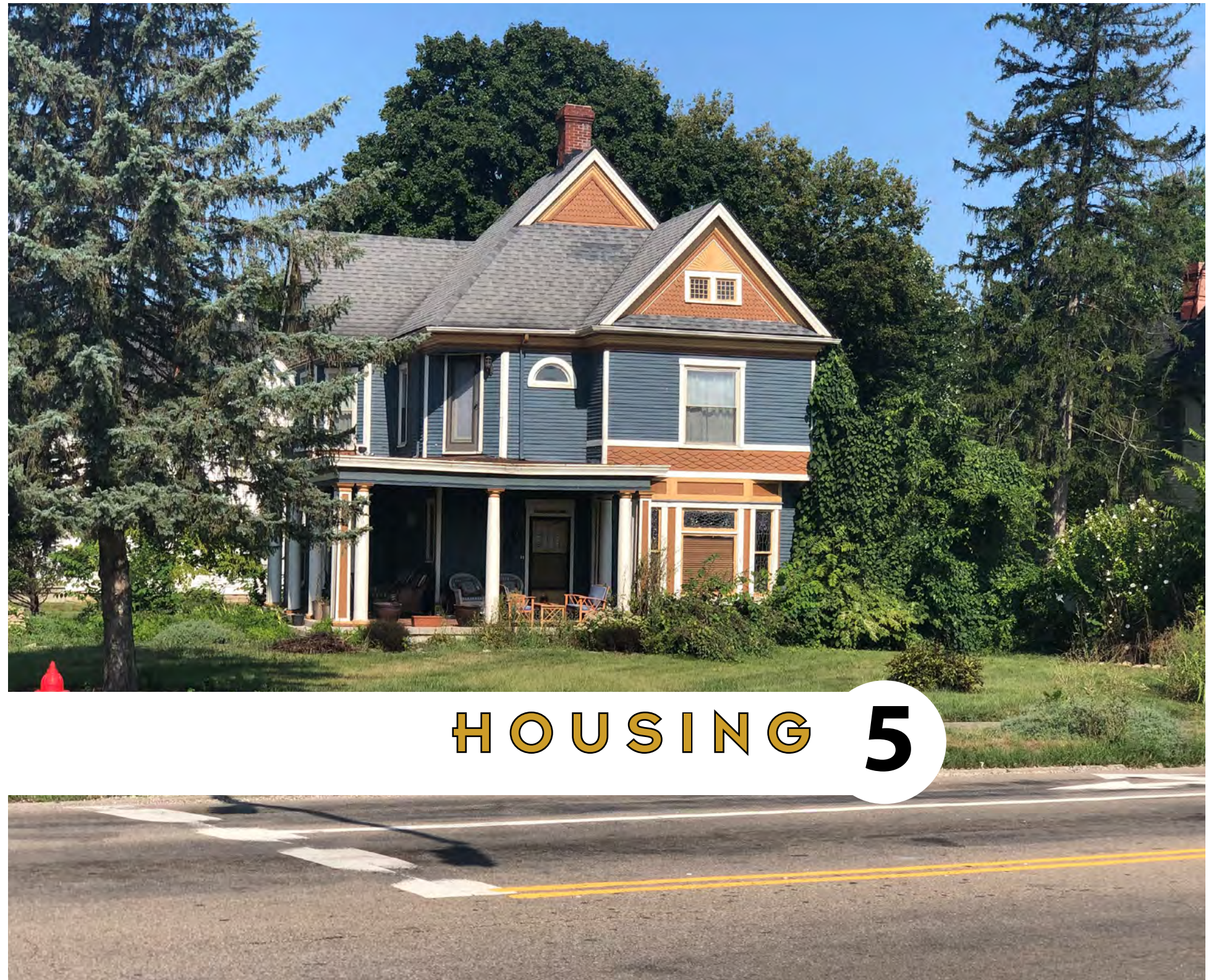
City of Franklin home within the Historic District
