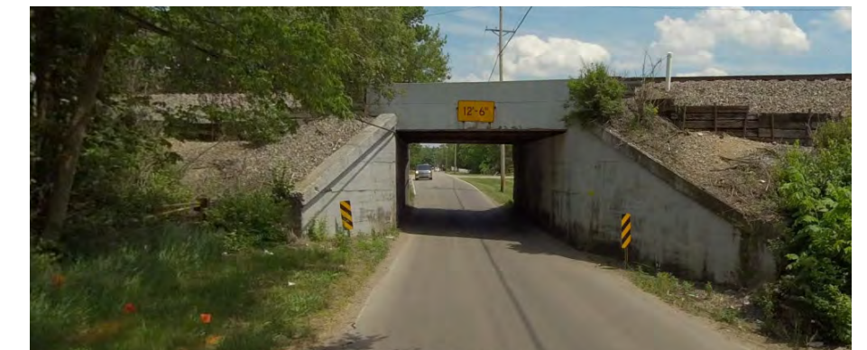
Railroad overpass along Franklin-Trenton Road
