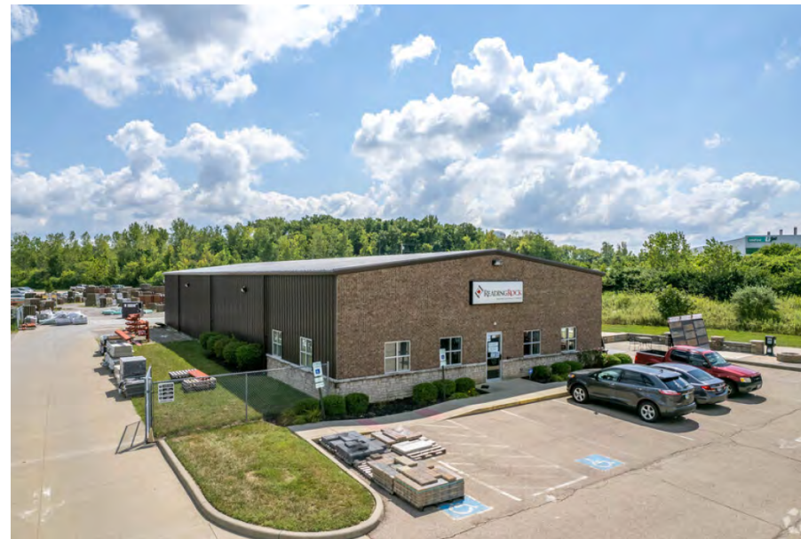
Industrial warehouse in Franklin
