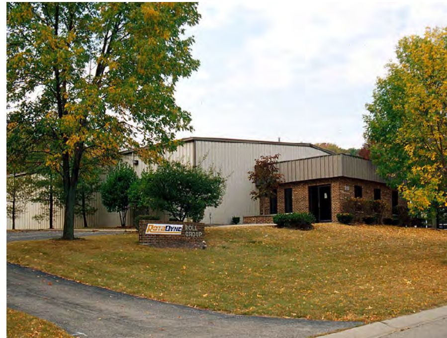
Industrial warehouse in Franklin
