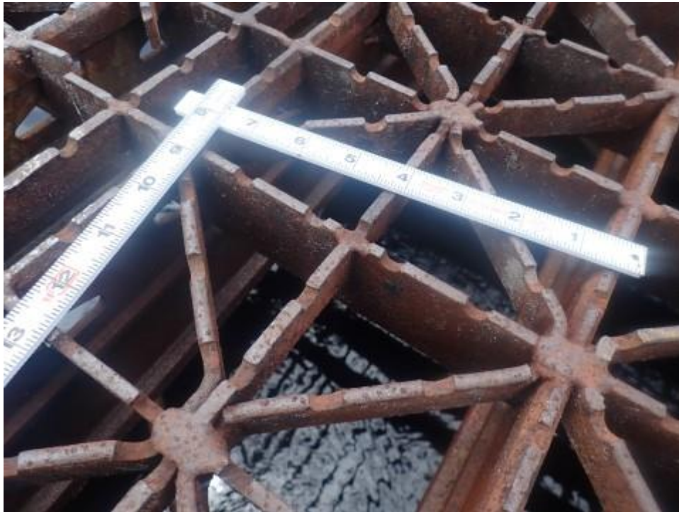
28 - Steel Deck - Open Grid (8516 - Painted Steel)
