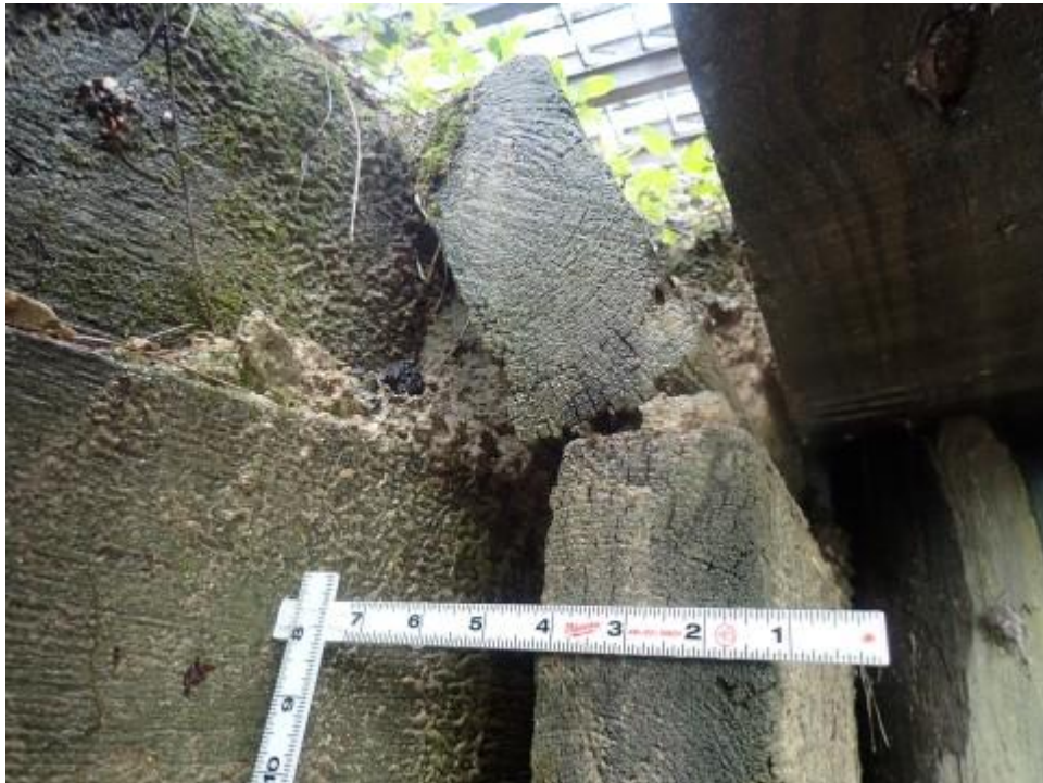
8395 - Timber Abutment Slope Protection
