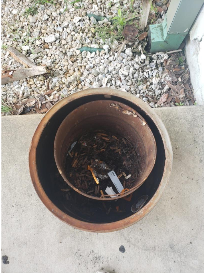
Cigarette receptacle bucket bottom completely rusted out and missing
