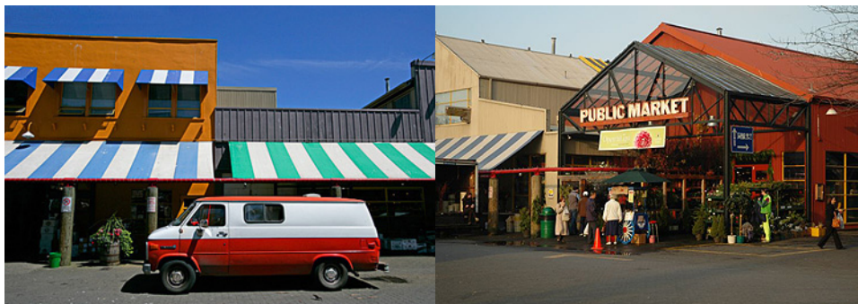
Examples of semi-industrial simplicity and informality. Simple materials and styles can have an authentic urban charm by emphasizing pedestrian-oriented building faces with glass, extensions, awnings, colors, signage, and well-kept planters. This kind of design is envisioned as having potential to create a fitting identity for key parts of the corridor.
