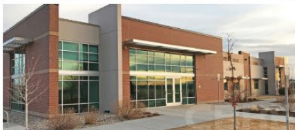
CBRE.com, Technology Parkway
