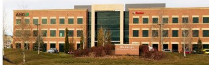
BryanConstruction.com, Harmony Corporate Center
