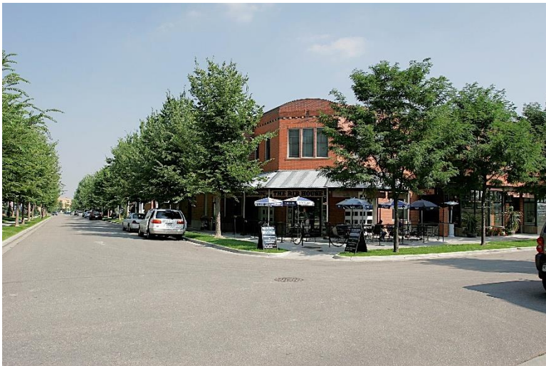
Building Fitted in and Brought to Streetfronts
