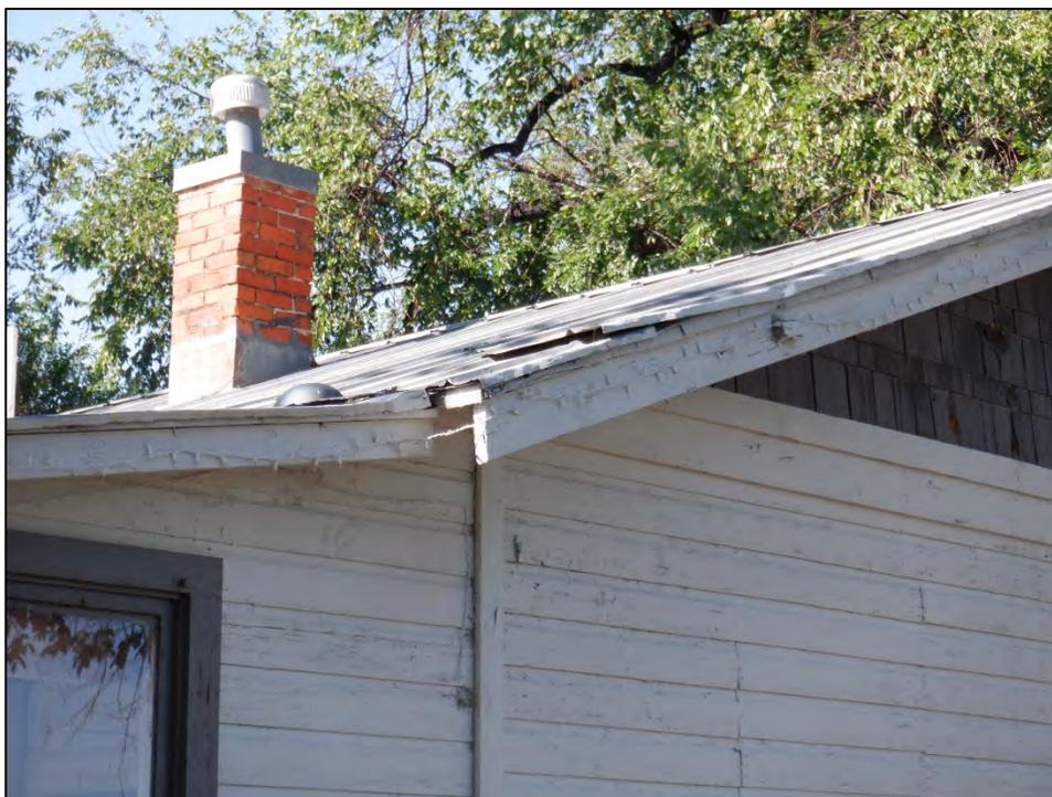
**Figure 8:** Feature 1, close up of loose roof panel, view southwest (Image #589, RLS 8/23/2022).
