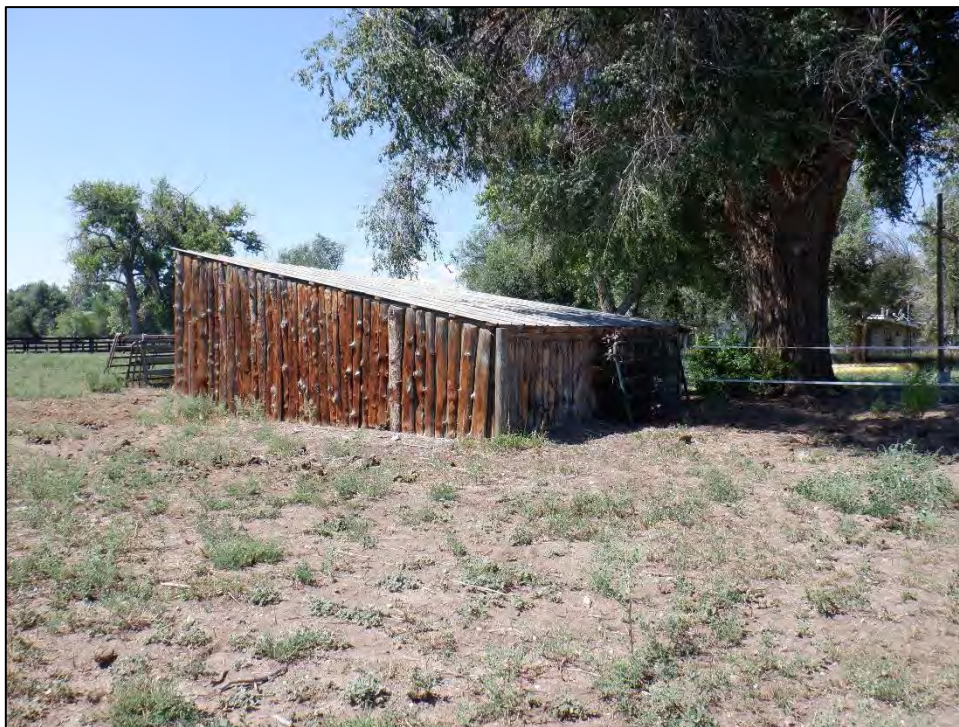
Figure 10: Feature 3, east and north elevations, view southwest (Image #649, RLS 8/23/2022).
