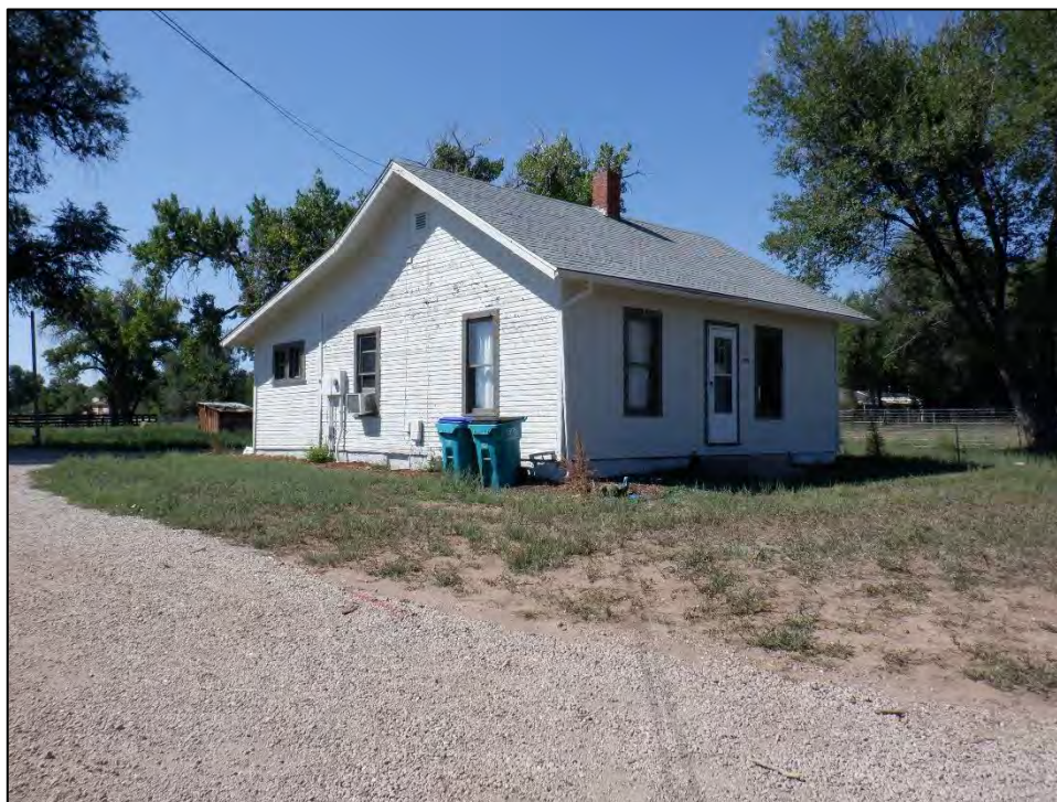
Figure 3: Feature 1, east and north elevations, view southwest (Image #636, RLS 8/23/2022).
