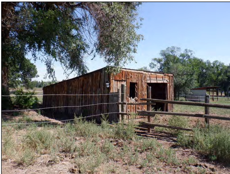
Figure 11: Feature 3, west and south elevations, view northeast (Image #651, RLS 8/23/2022).
