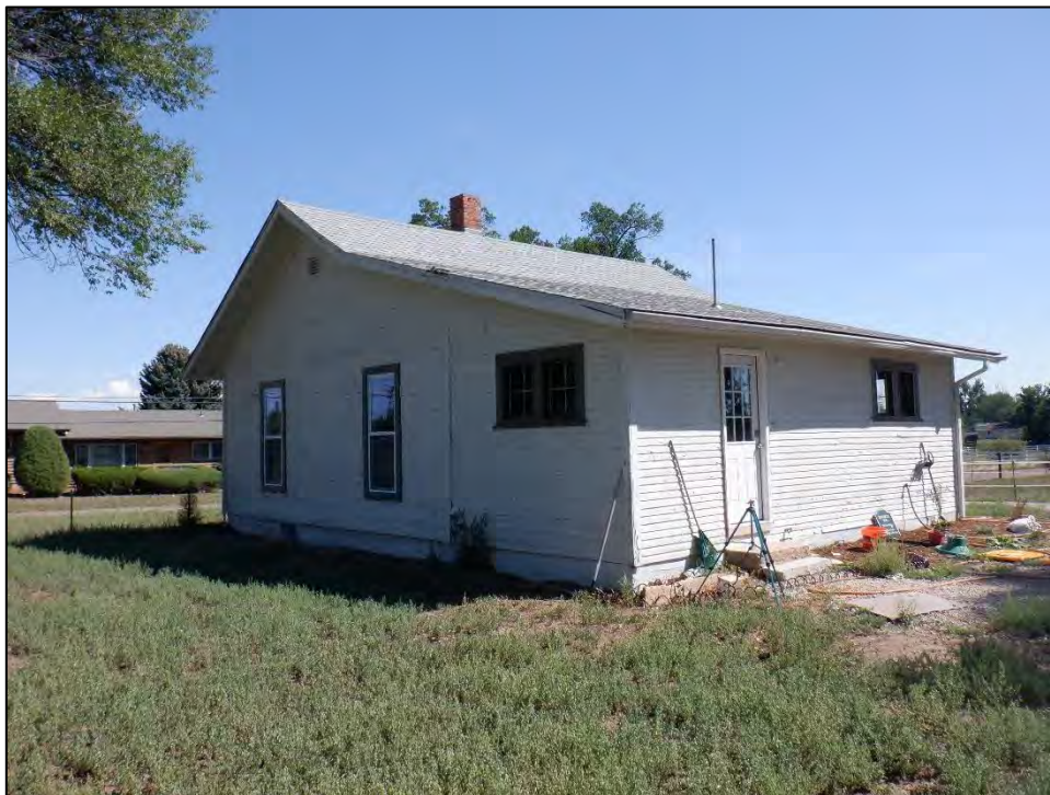
Figure 5: Feature 1, west and south elevations, view northeast (Image #638, RLS 8/23/2022).
