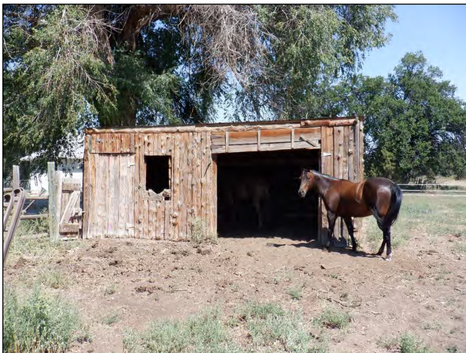
Figure 9: Feature 3, south elevation, view north (Image #647, RLS 8/23/2022).
