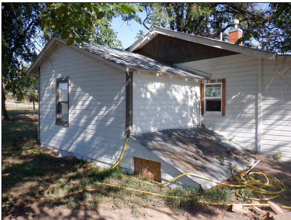
Figure 7: Feature 1, close-up of south elevation, view northwest (Image #586, RLS 8/23/2022).
