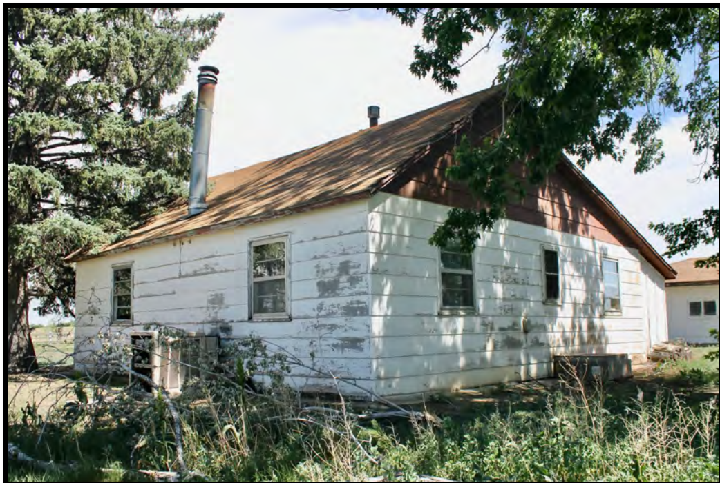
House, View to the Southeast
