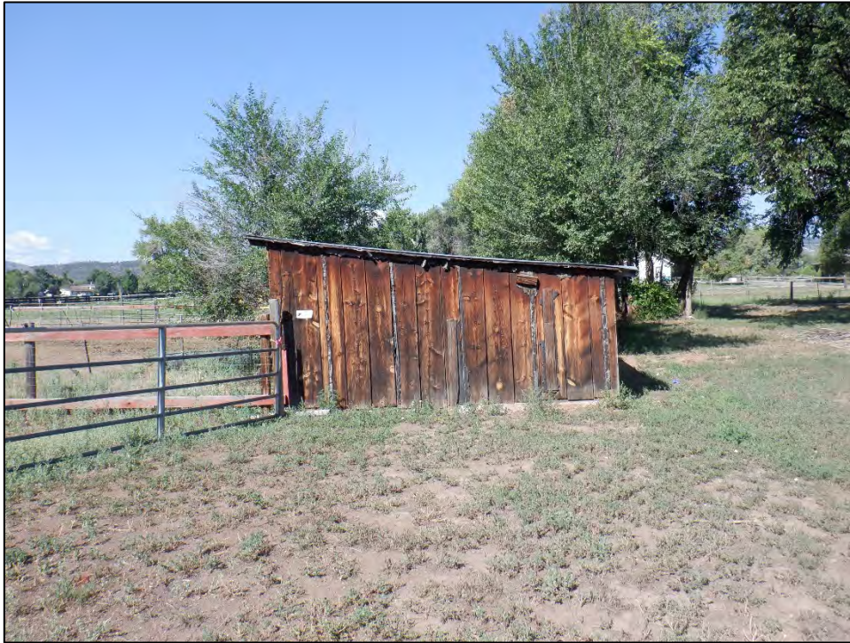
Figure 13: Feature 2, east elevation, view west (Image #606, RLS 8/23/2022).
