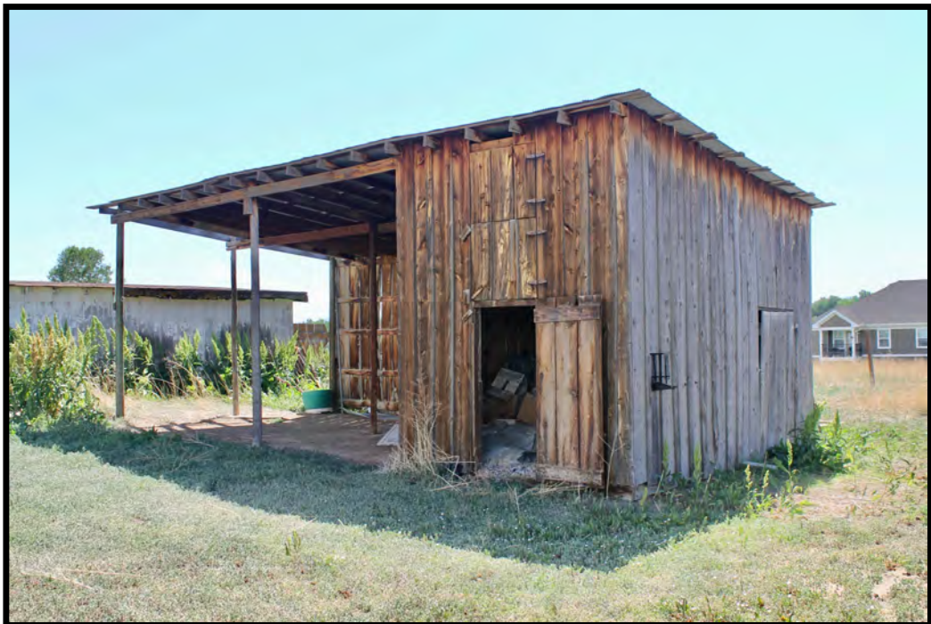
Hay Shed, View to the Southwest
