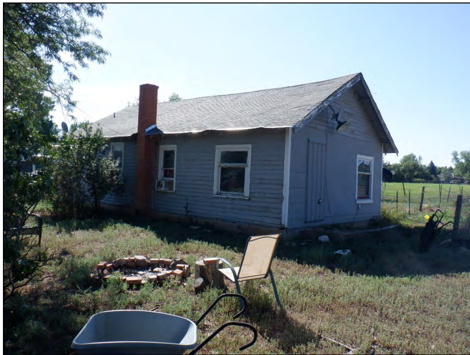
Figure 4: Feature 1, north and west elevations, view southeast (Image #614, RLS 8/23/2022).
