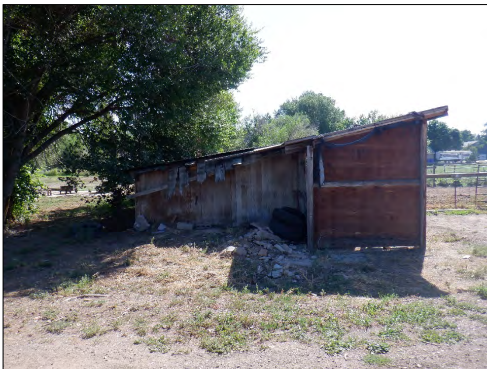
Figure 10: Feature 2, west elevation, view east (Image #600, RLS 8/23/2022).
