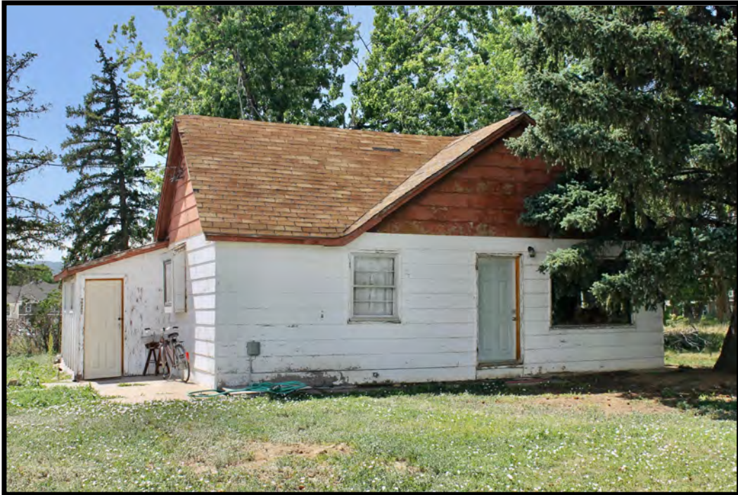
House, View to the Northwest
