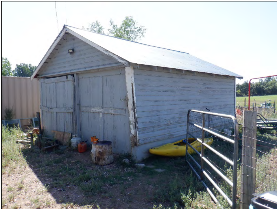
Figure 8: Feature 2, west and north elevations, view southeast (Image #626, RLS 8/23/2022).
