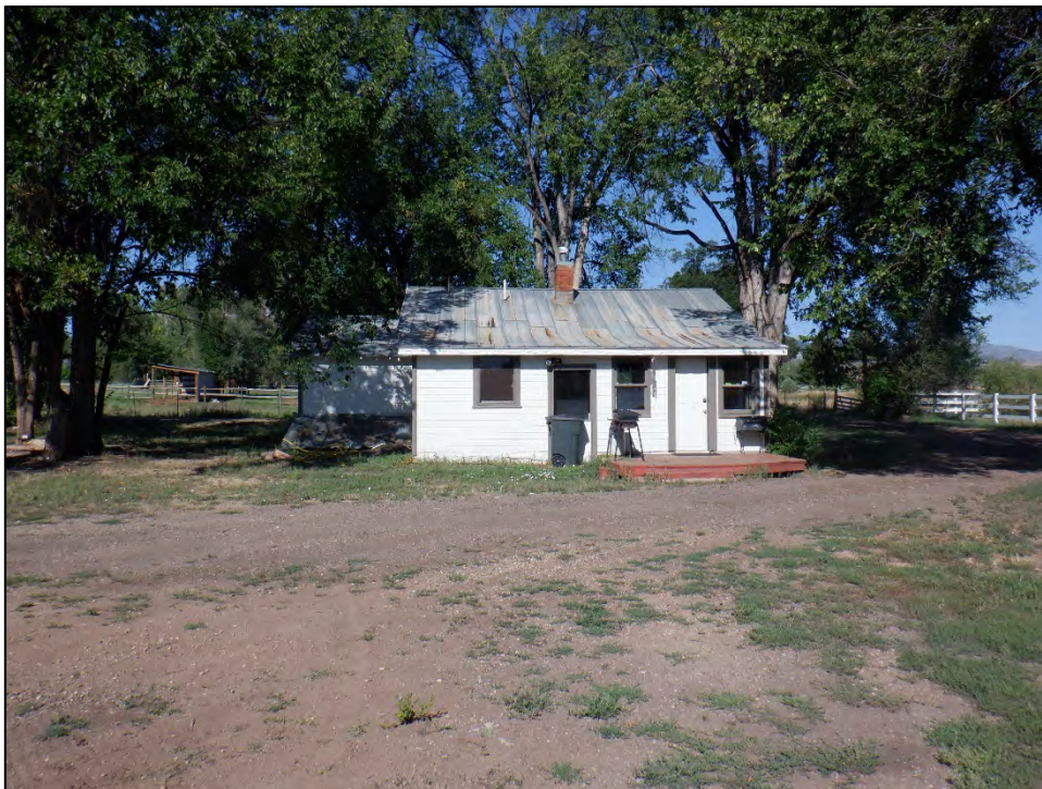
Figure 2: Feature 1, east elevation, view west (Image #578, RLS 8/23/2022).
