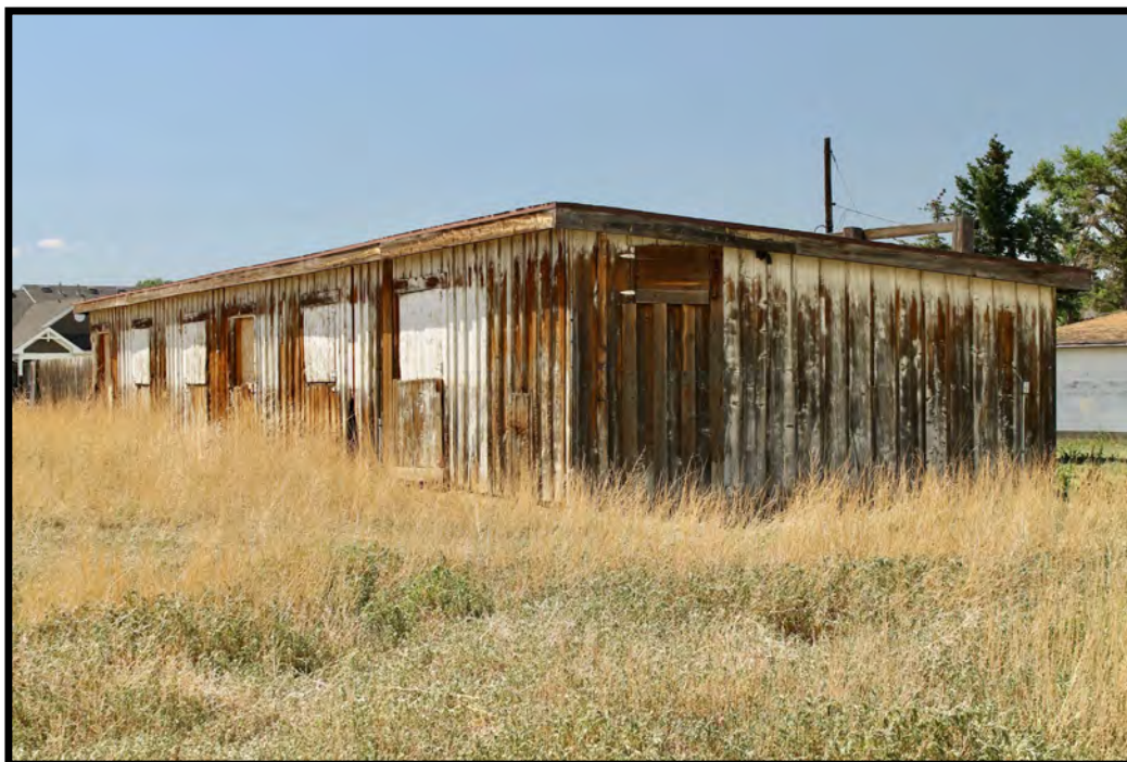
Horse Barn, View to the Northwest
