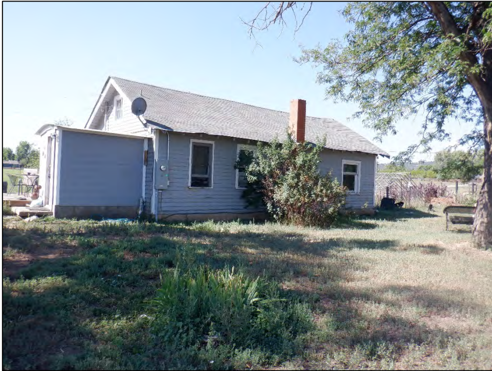
Figure 3: Feature 1, north elevation, view southwest (Image #612, RLS 8/23/2022).
