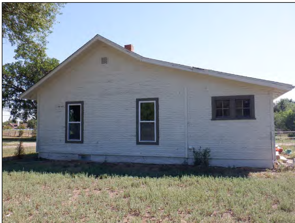
Figure 6: Feature 1, west elevation, view east (Image #639, RLS 8/23/2022).
