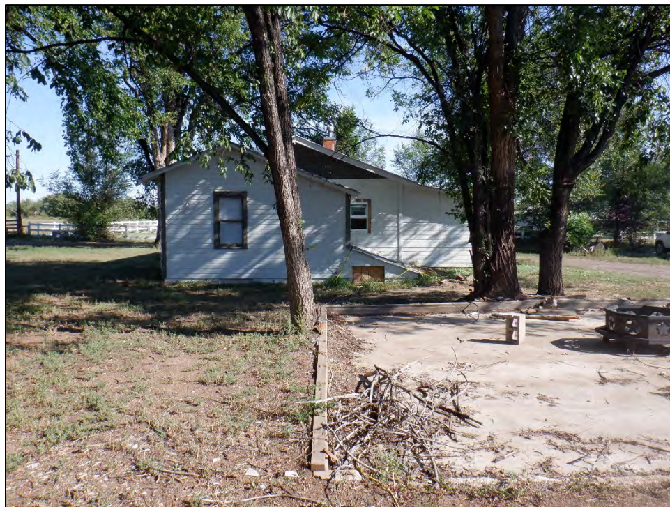
Figure 6: Feature 1, south elevation, view north (Image #584, RLS 8/23/2022).
