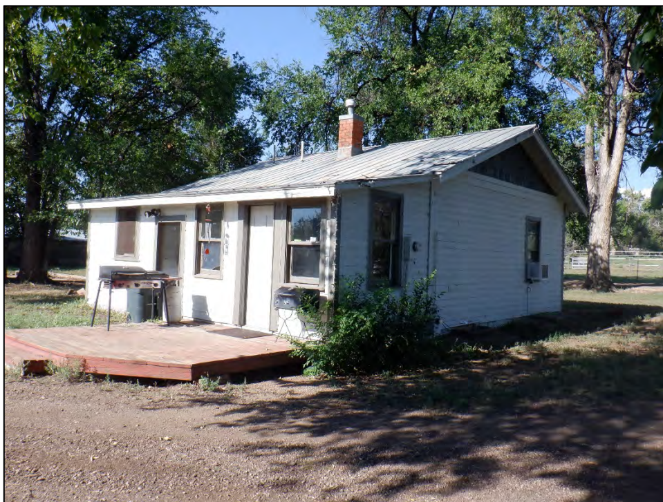
Figure 3: Feature 1, east and north elevations, view southwest (Image #679, RLS 8/23/2022).
