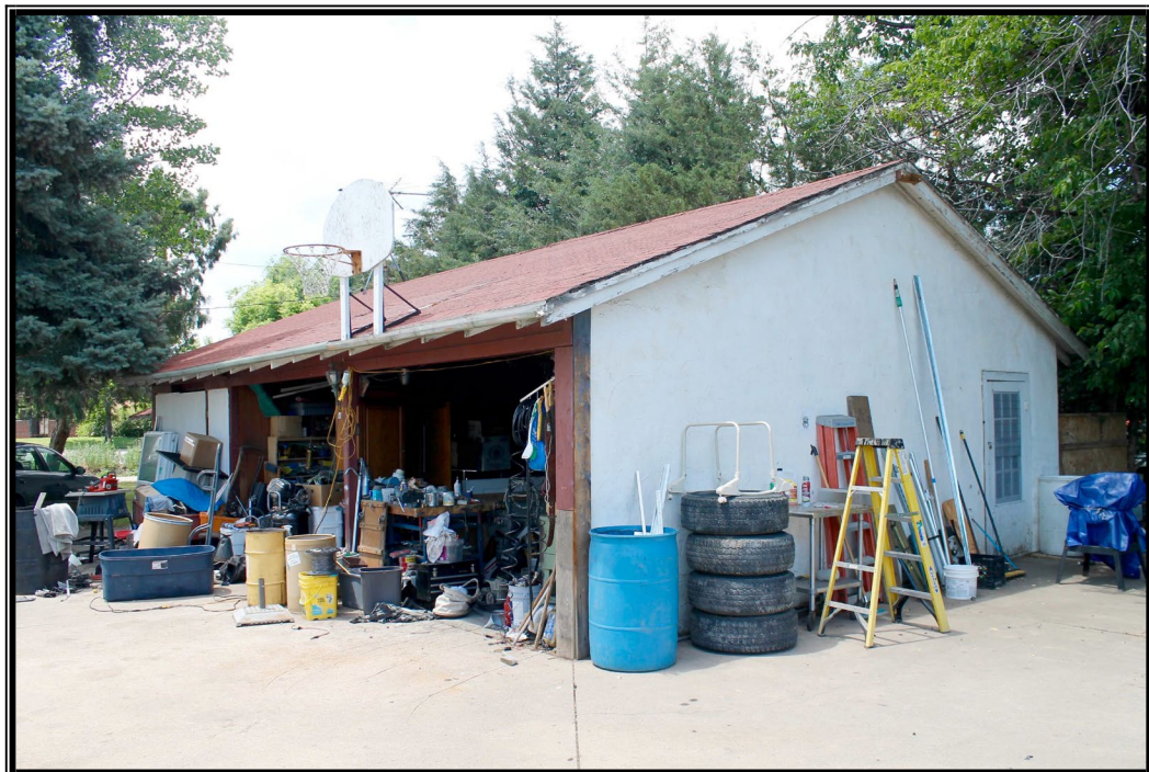
Garage, View to the Northwest
