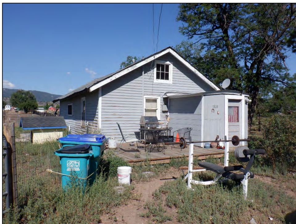
Figure 2: Feature 1, south and east elevations, view northwest (Image #610, RLS 8/23/2022).
