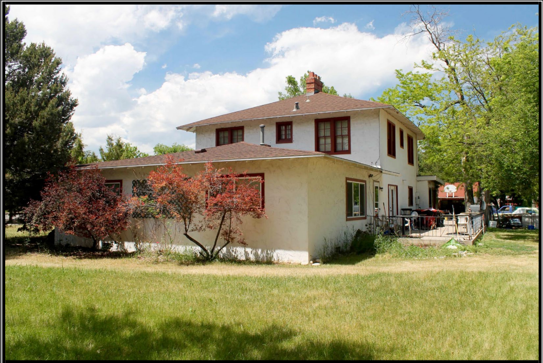
Main House, View to the Northwest
