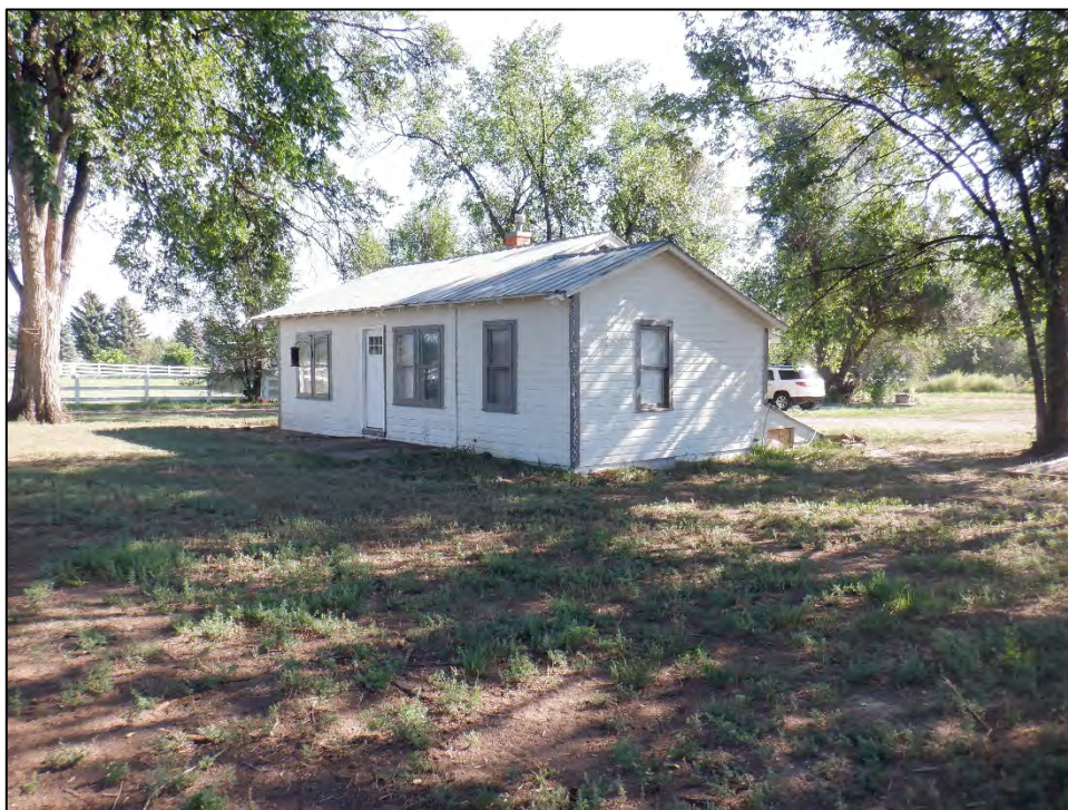
Figure 5: Feature 1, west and south elevations, view northeast (Image #583, RLS 8/23/2022).
