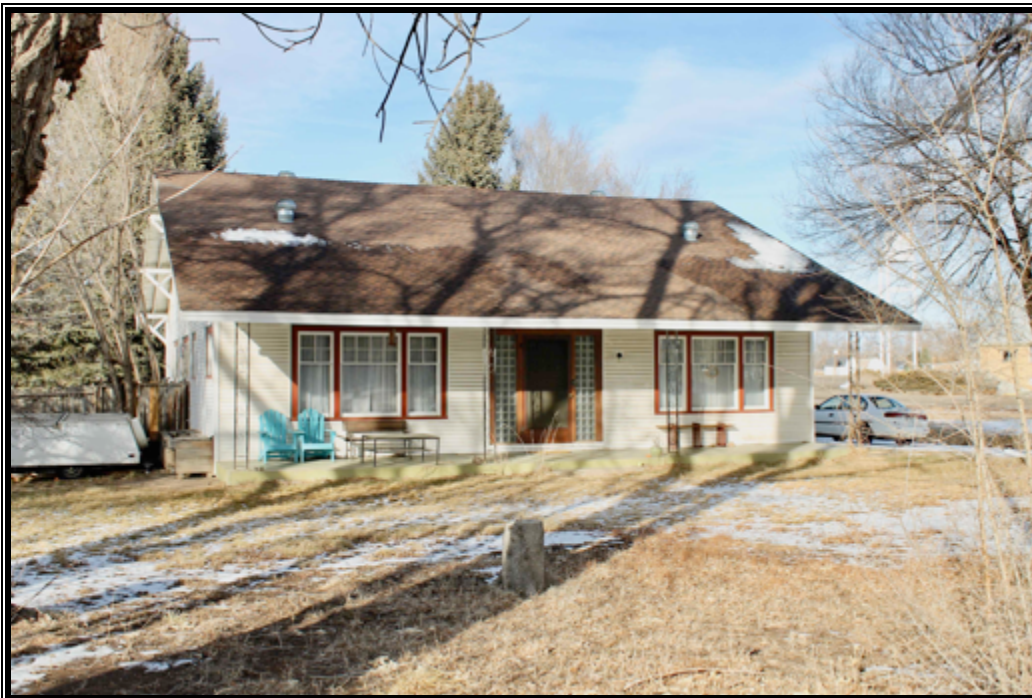
View of the House View to the Northeast
