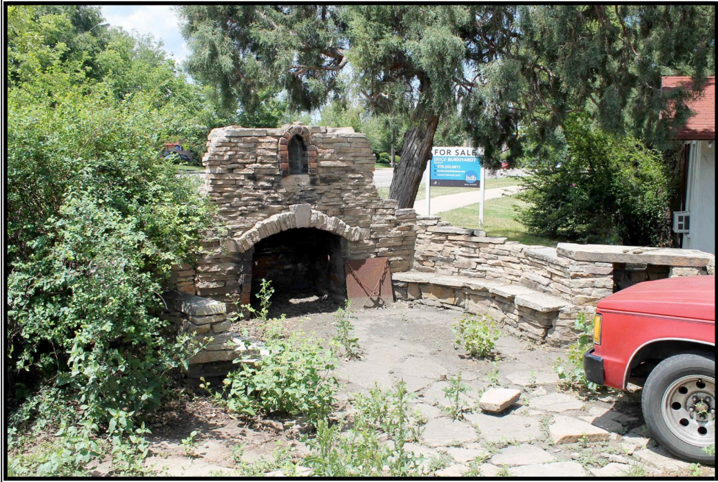
Fireplace and Terrace, View to the Northwest
