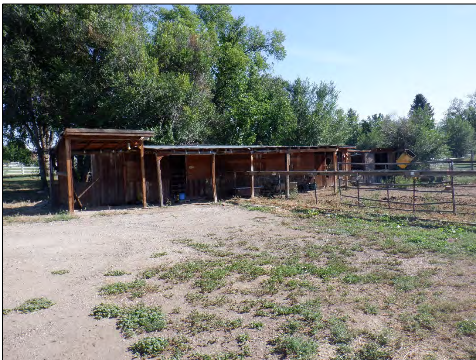
Figure 9: Feature 2, south elevation, view northeast (Image #597, RLS 8/23/2022).
