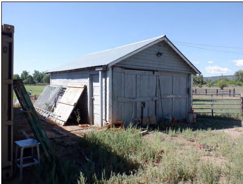
Figure 7: Feature 2, east and north elevations, view southwest (Image #624, RLS 8/23/2022).
