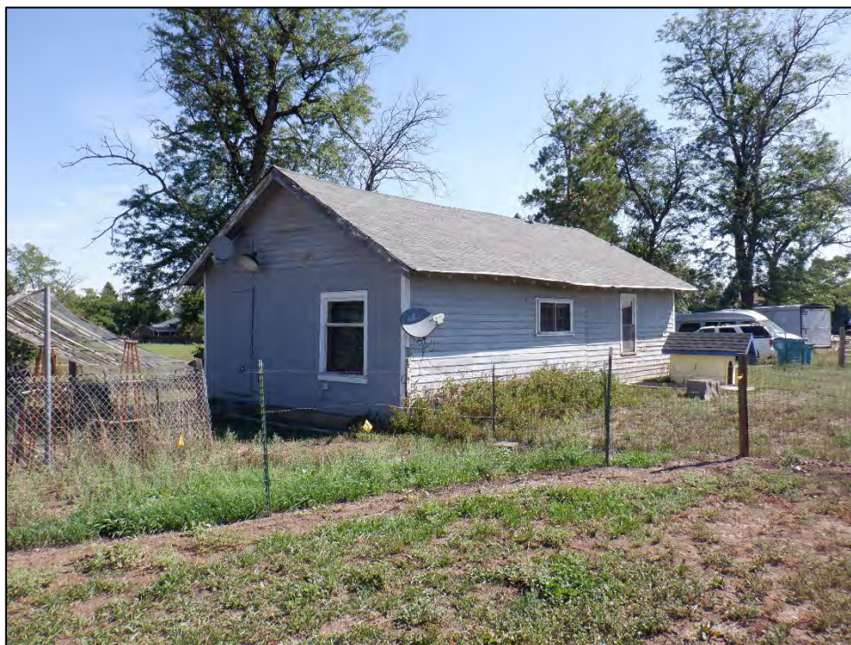
Figure 5: Feature 1, west and south elevations, view northeast (Image #616, RLS 8/23/2022).
