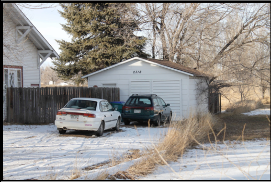
View of the Garage View to the Northwest
