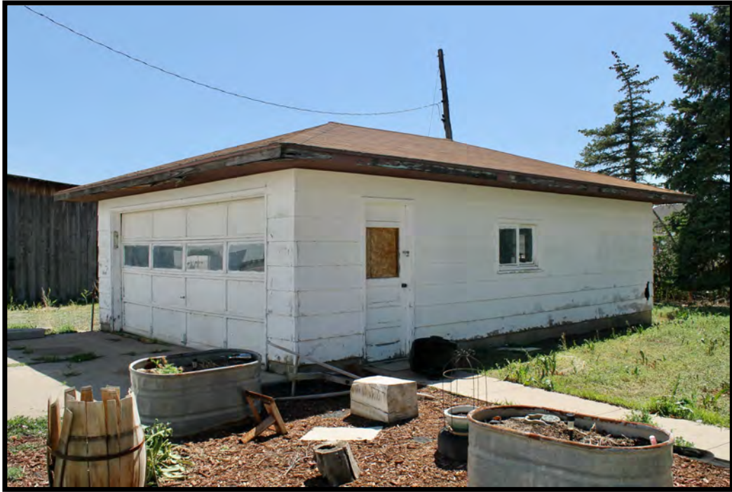
Garage, View to the Southwest
