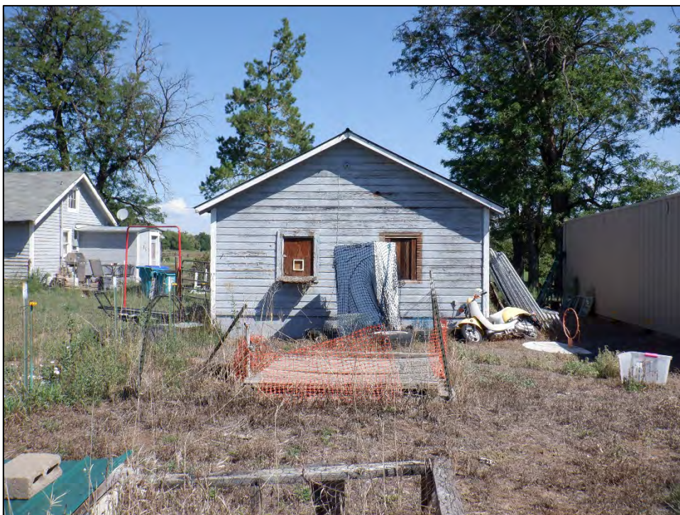
Figure 8: Feature 2, south elevation, view north (Image #628, RLS 8/23/2022).
