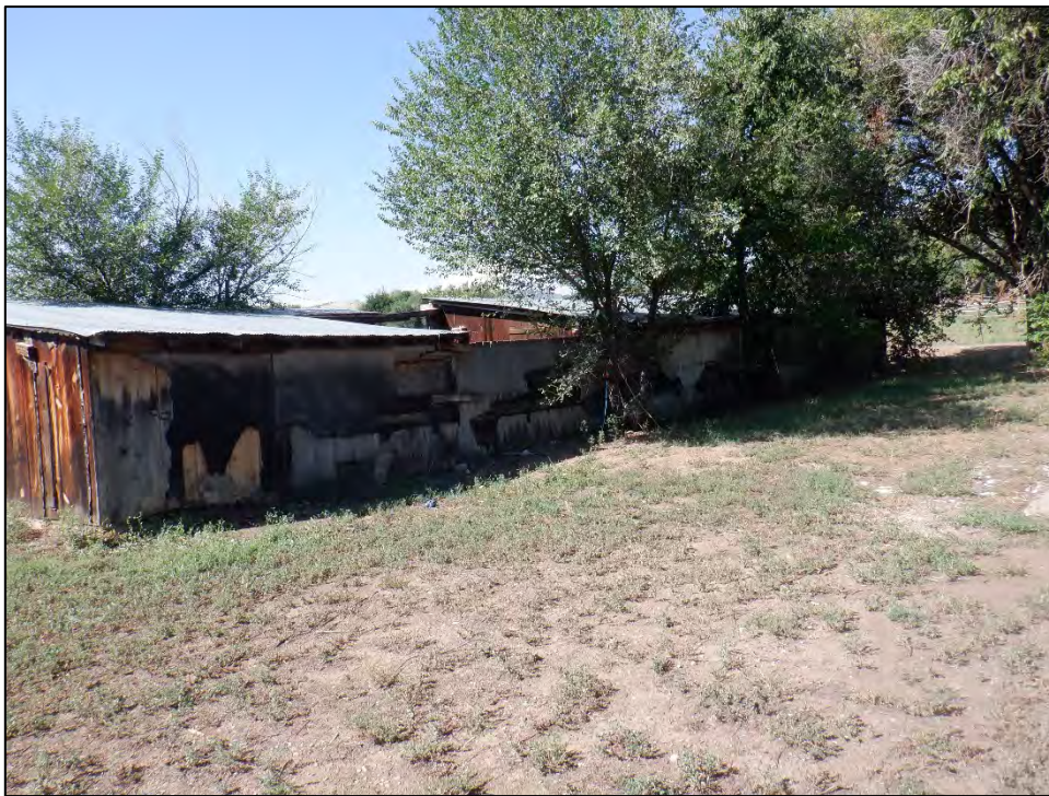
Figure 12: Feature 2, south elevation, view southwest (Image #605, RLS 8/23/2022).
