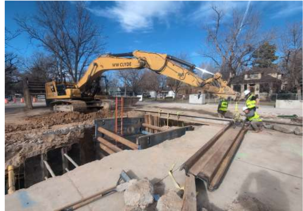
“Open Cut” Pipe Installation
