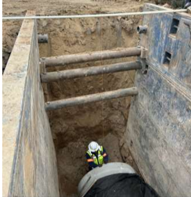
“Open Cut” Pipe Installation
