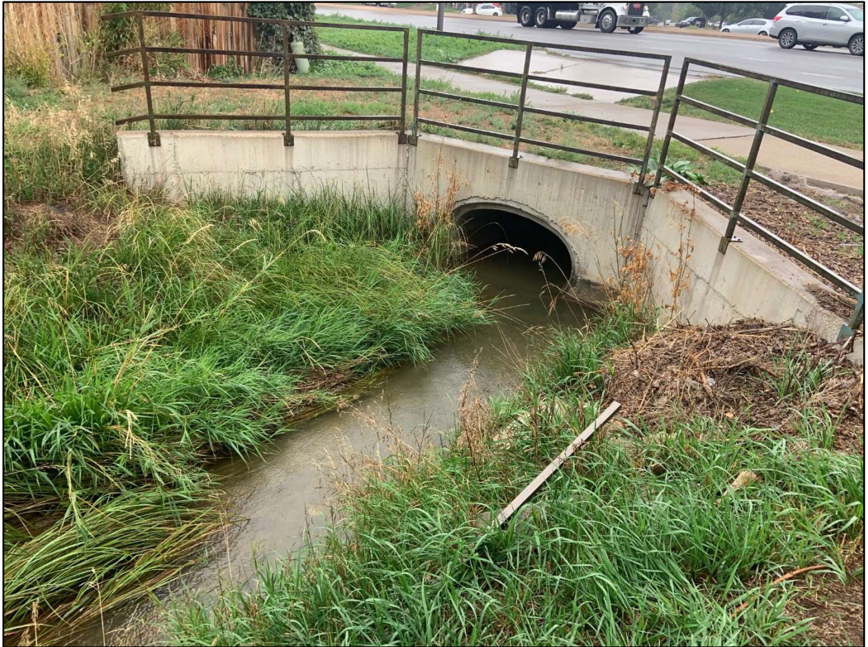
Photo 14. Timberline and Harmony: Dixon Canyon Lateral entering a culvert on the west side of Timberline Road at the intersection with Harmony Road. Banks were heavily vegetated with a mixture of upland and wetland vegetation.
