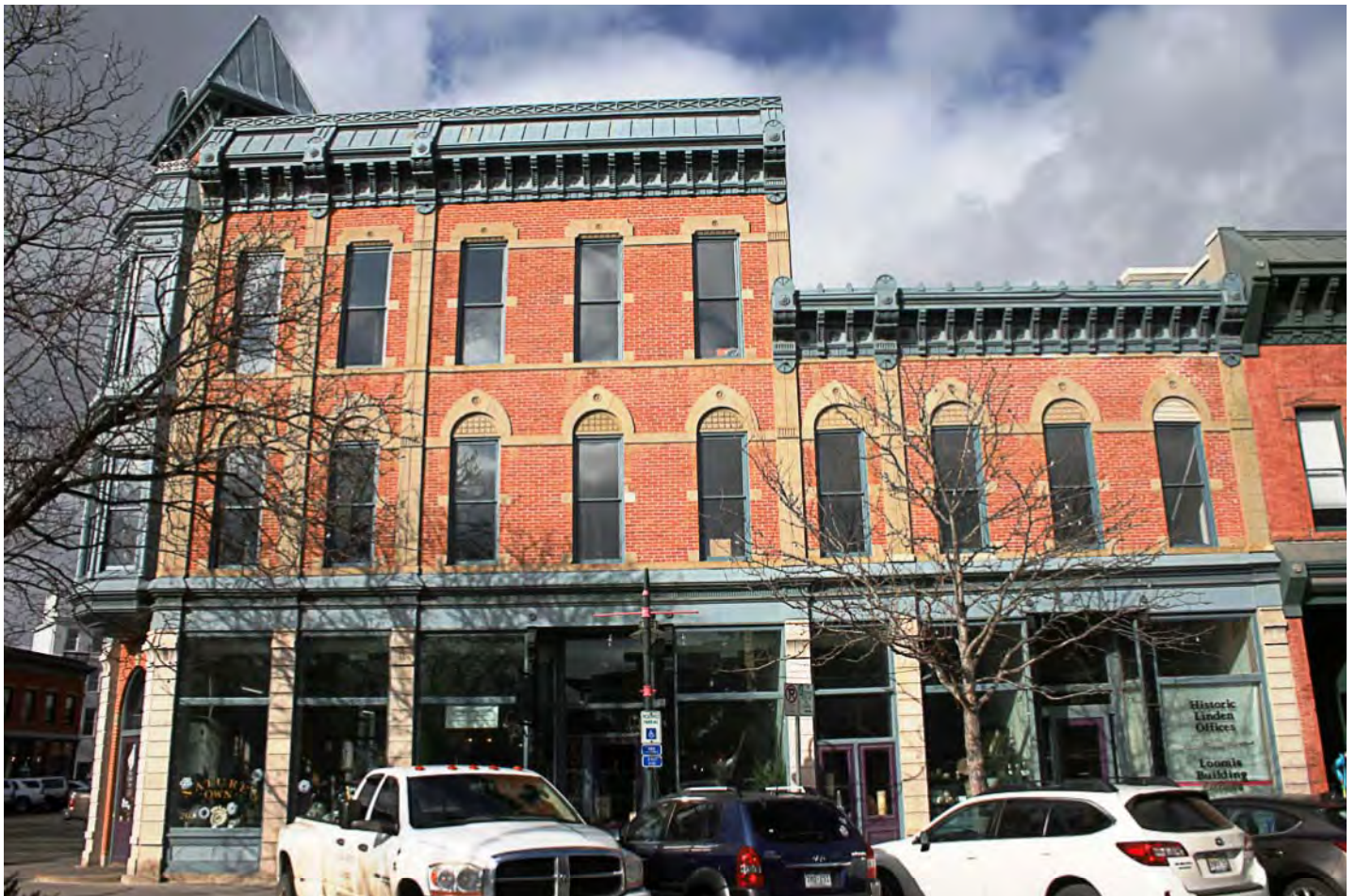
Linden Street Elevation_Faces Southeast
