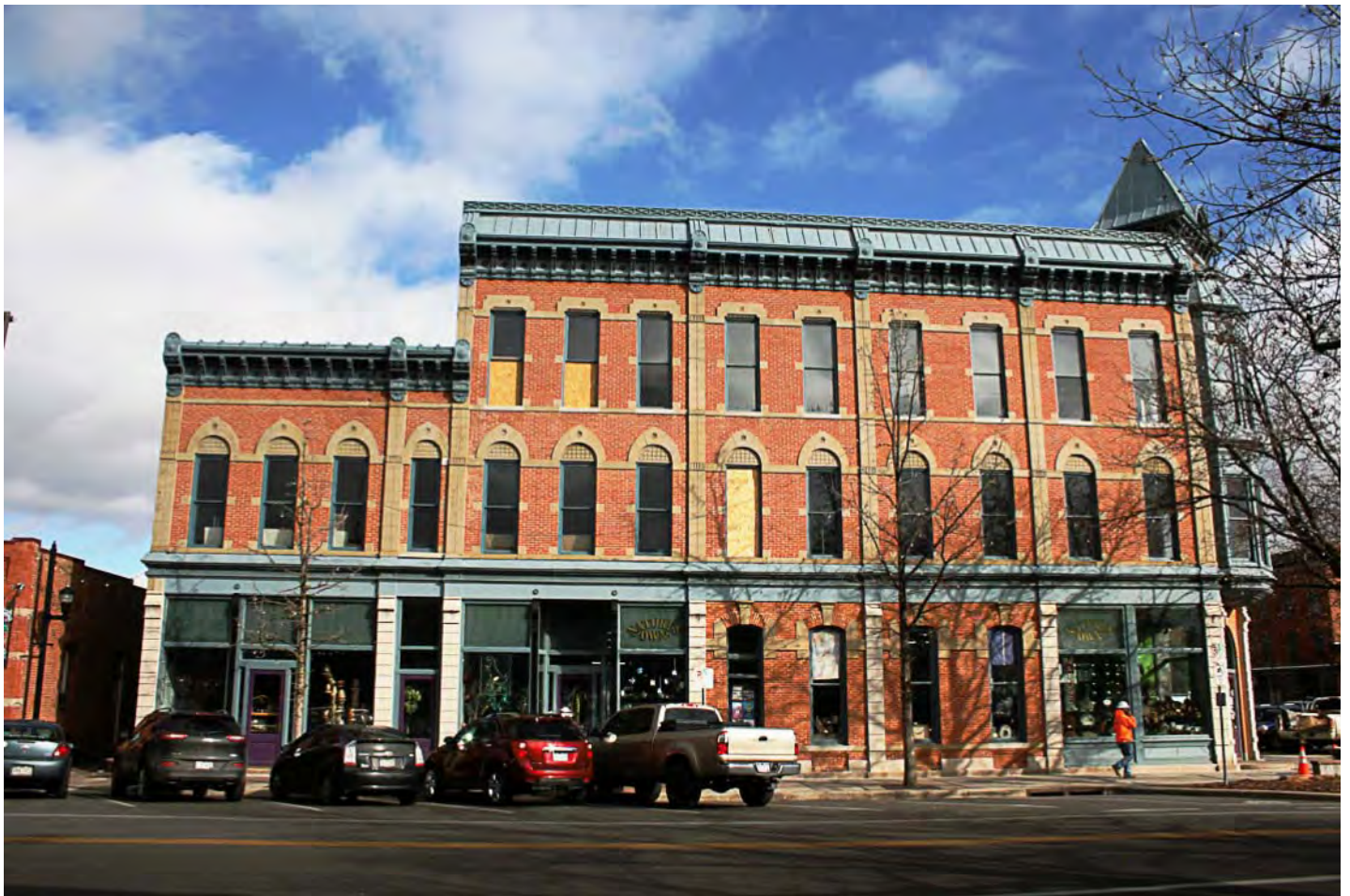
Walnut Street Elevation, Faces Southwest
