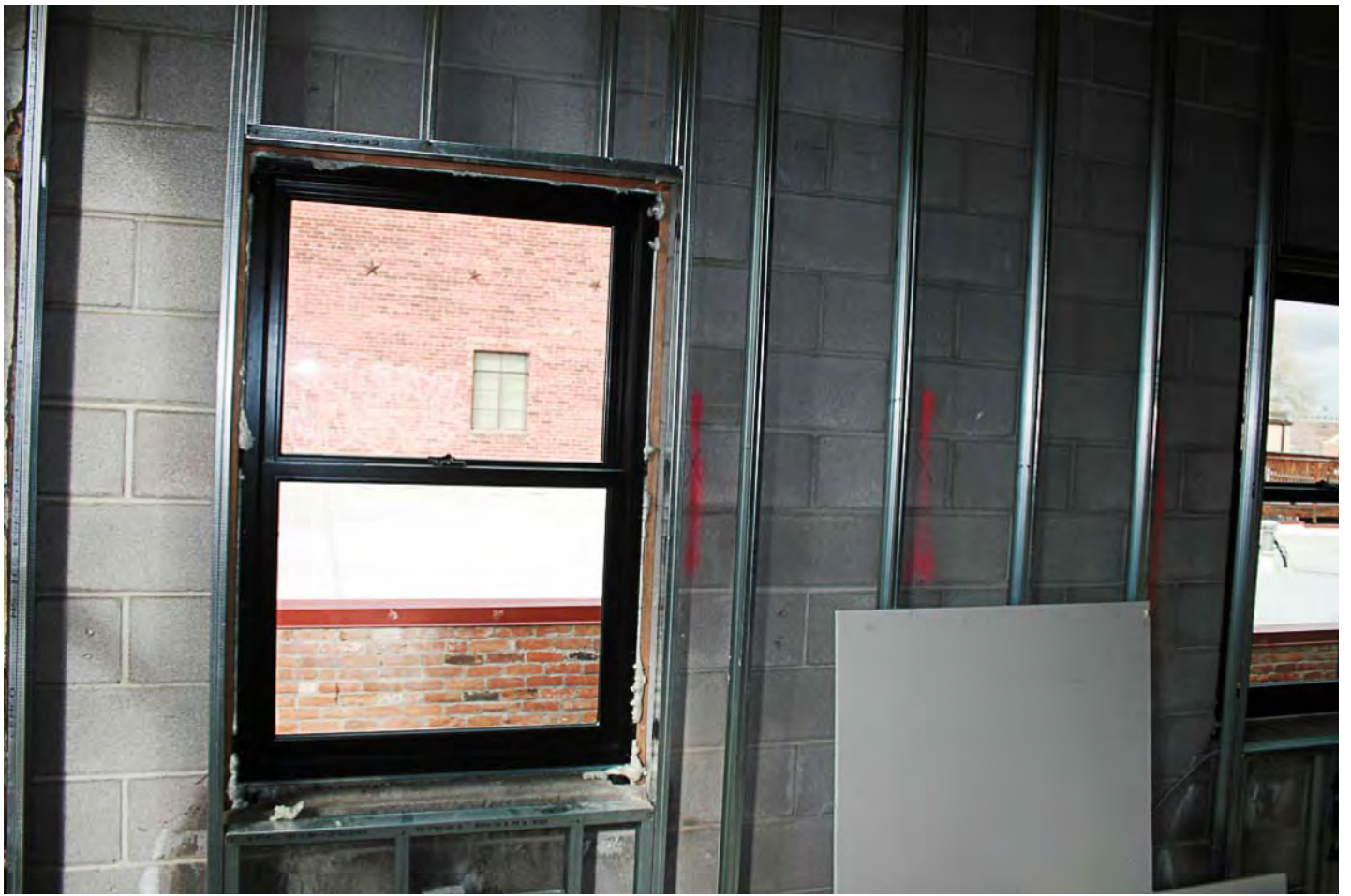
Replacement windows_Northwest elevation_Alley
