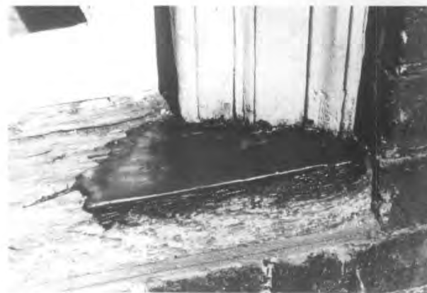
Figure 5. This illustrates a two-part epoxy patching compound used to fill the surface of a weathered sill and rebuild the missing edge. When the epoxy cures, it can be sanded smooth and painted to achieve a durable and waterproof repair. Photo: John H. Myers
