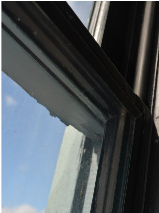
Replaced Check Rail
