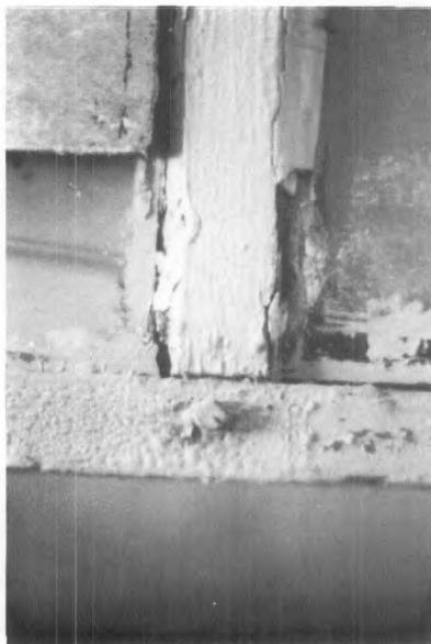
Figure 4a. The following series of photographs of the repair of a historic double-hung window use a unit which is structurally sound but has many layers of paint, some cracked and missing putty, slight separation at the joints, broken sash cords, and one cracked pane. Photo: John H. Myers
