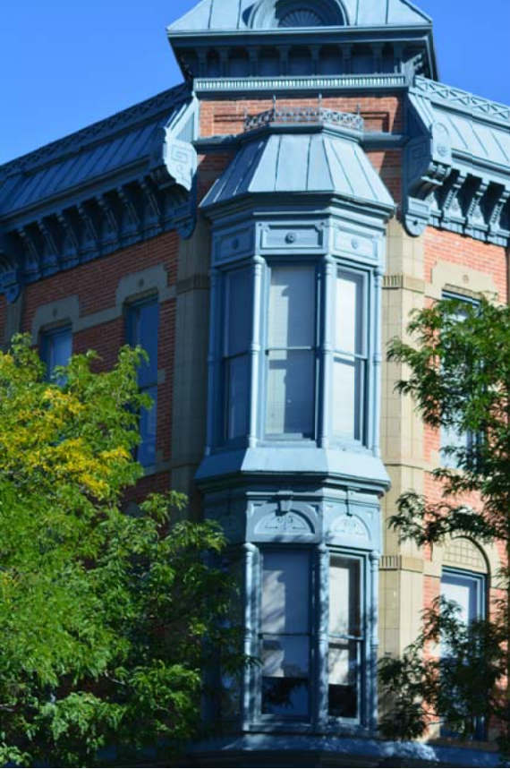
South East Corner
