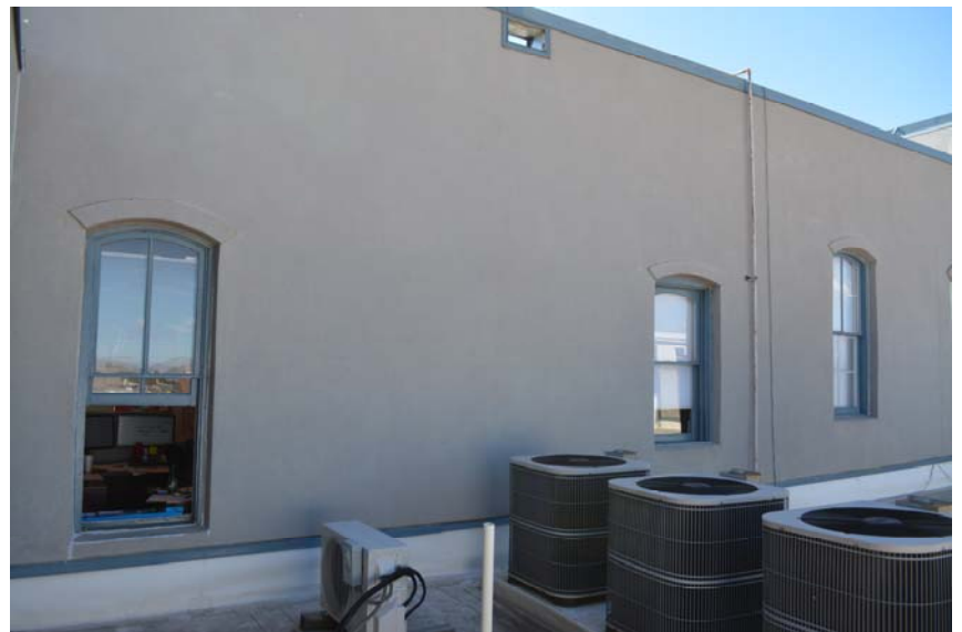
Third Floor West Windows
