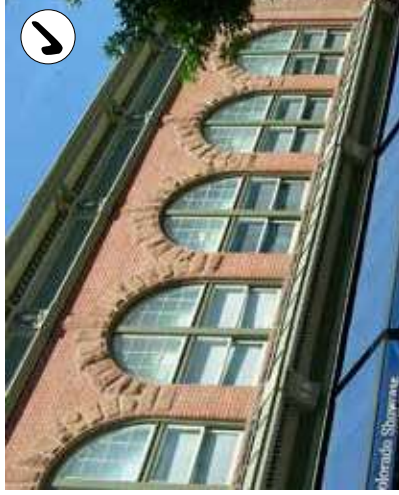
After rehabilitation: repaired windows.
