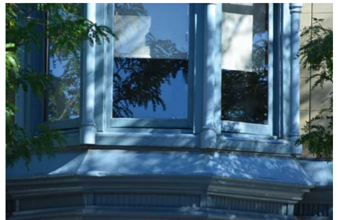
3rd Floor Corner Sill
