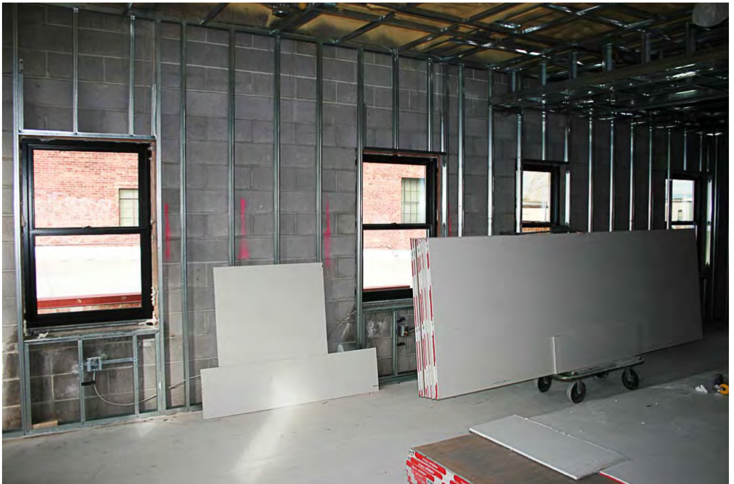
Replacement windows_Northwest elevation_Alley 2
