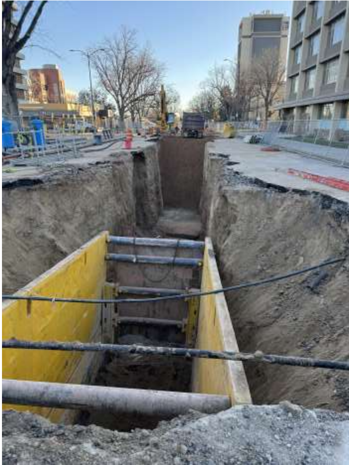
“Open Cut” Pipe and Inlet Installations
