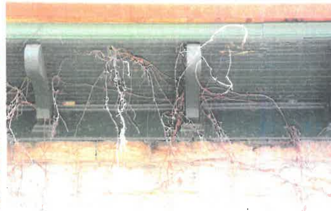
REFURBISH SOFFITS REMOVE IVY
