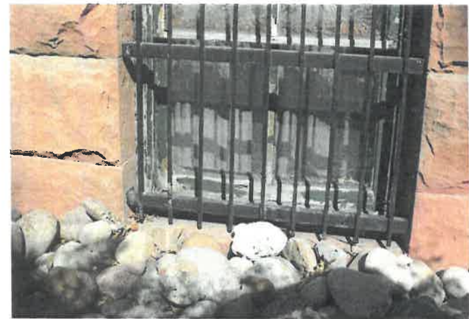
REFURBISH WINDOW FRAMES
