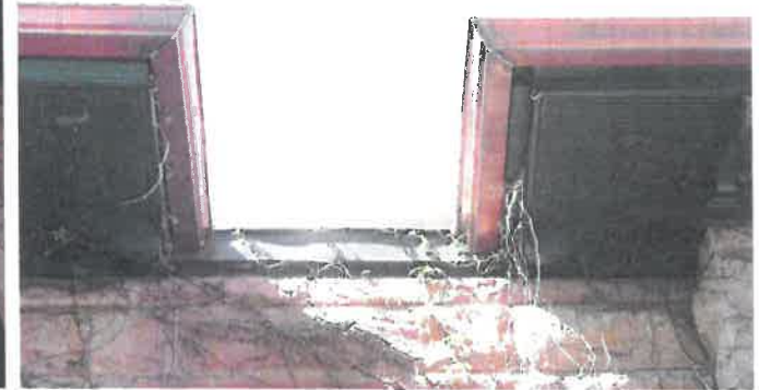
REFURBISH SOFFITS REMOVE IVY
